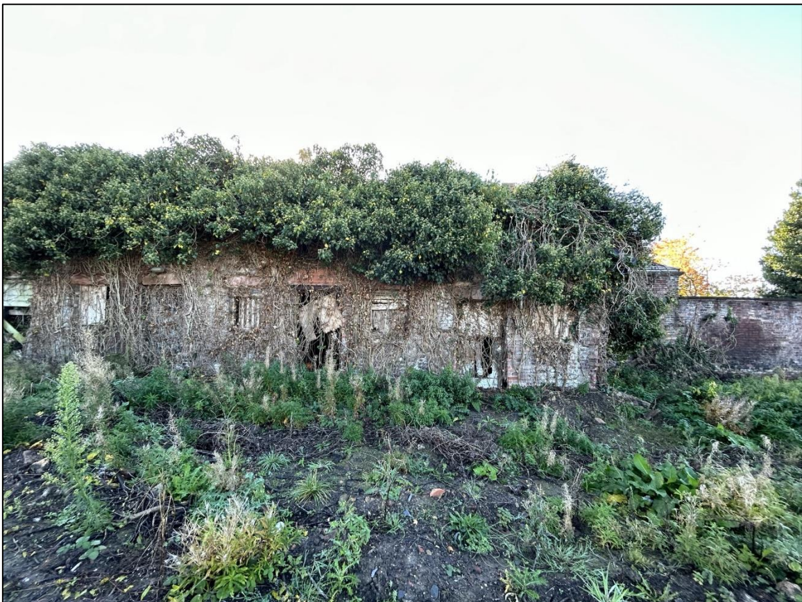
Plate 6 – Northern elevation of B2
