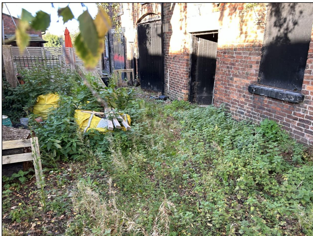
Plate 11 – Cobbled area with emergent vegetation growth
