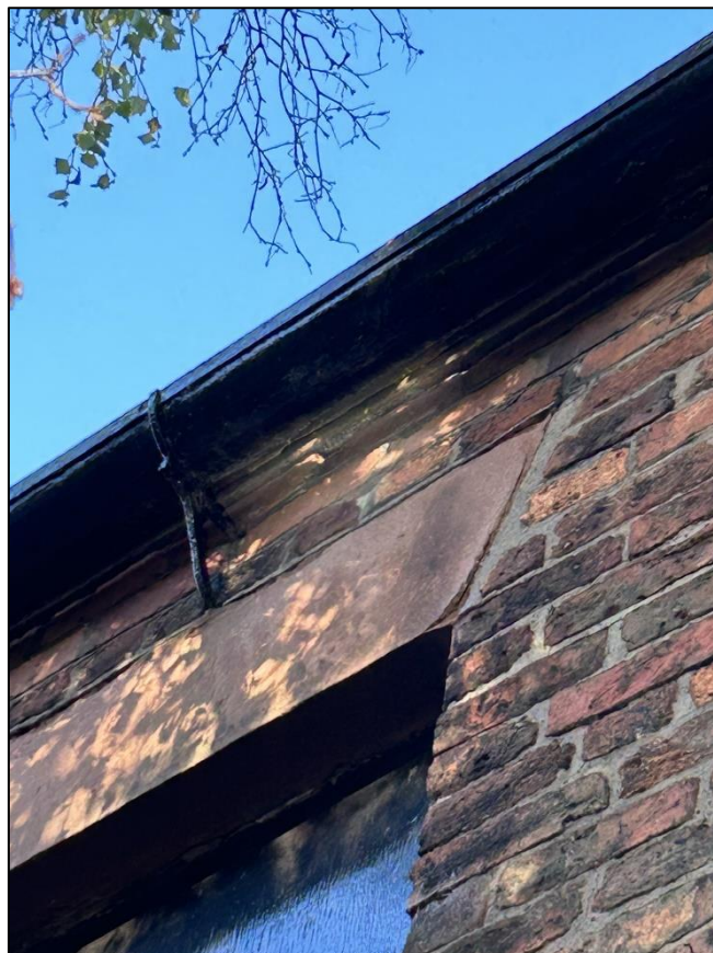
Plate 4 – Indicative entry points at wall plate level on the southern elevation
