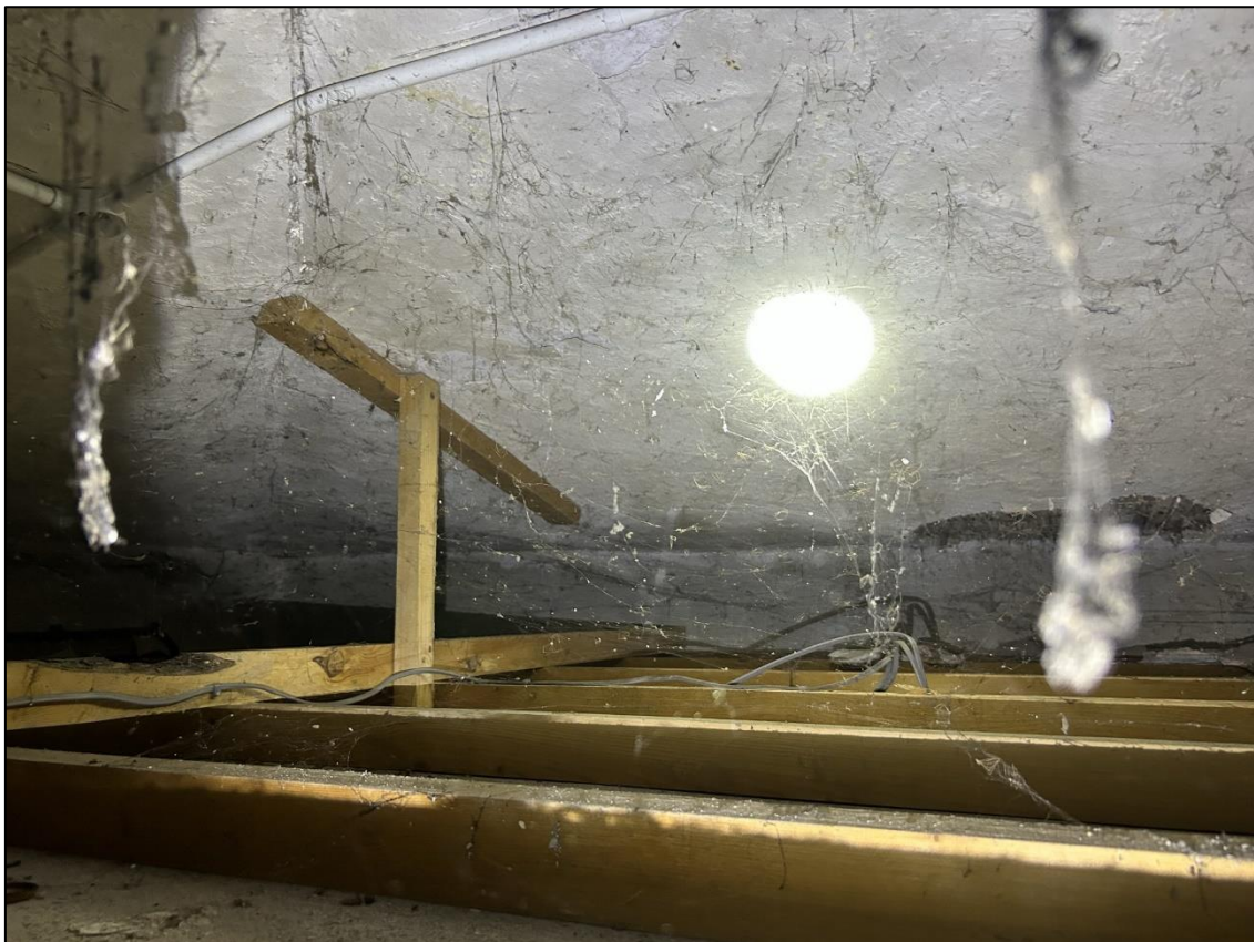
Plate 8 – Loft space above the single storey region of B2
