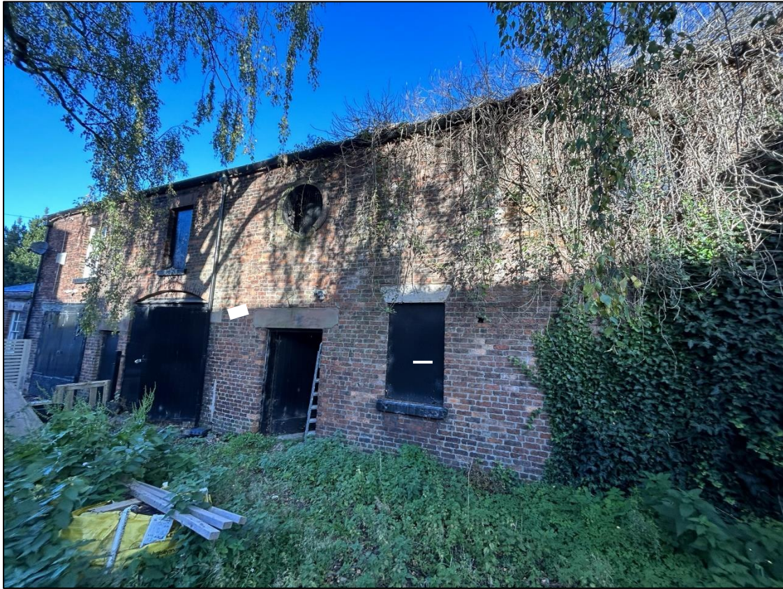
Plate 1 – The southern elevation of Building B2, The Stable Block, Grade II Listed
