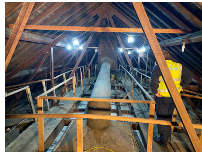
The roof space above the main auditorium
