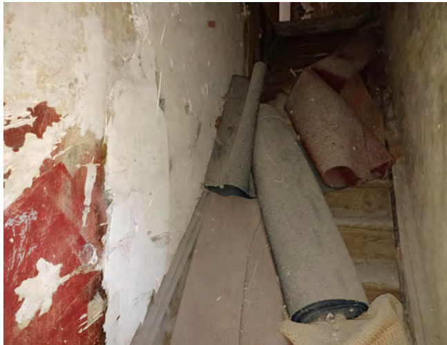
A mid-late 19th century staircase between first and second floors
