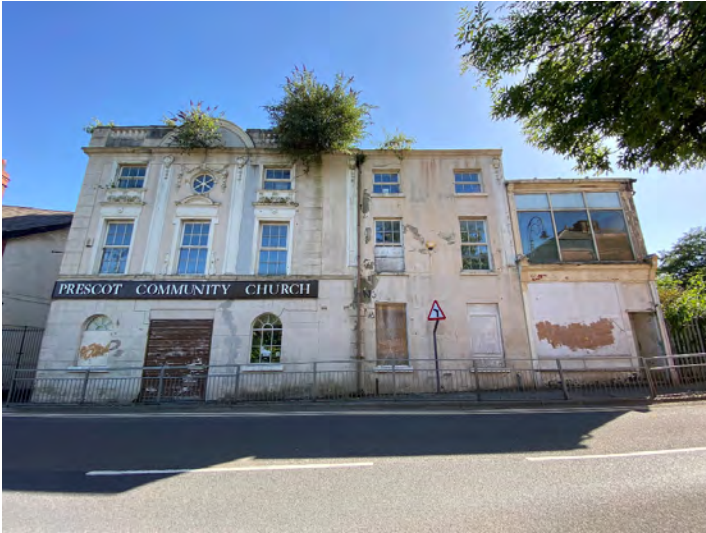
The building as viewed from the road
