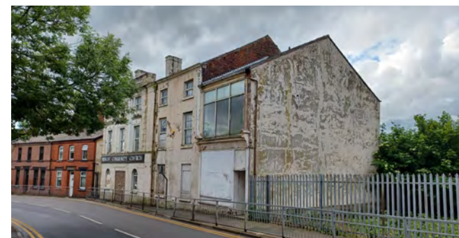
The building with the vacant plot to the west negatively contributing to the setting of the site
