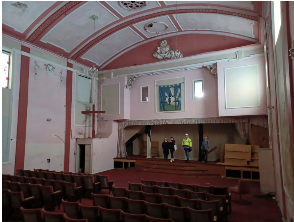
The auditorium today with the boxing to the left a later alteration to install a staircase and room behind.
