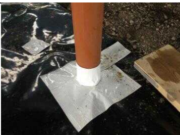
Typical pipe detail to core area 1.
