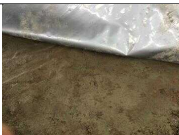
Membrane installed upon a sand blinding substrate within Core Area 2.
