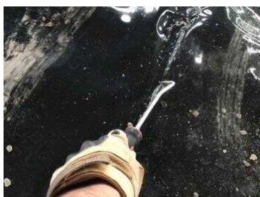
Testing to the welded lap joint to core area 2.
