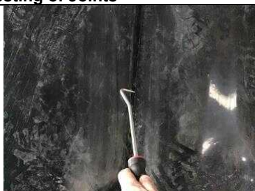
Welded lap joint testing
