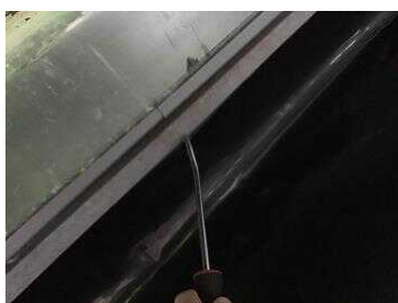
Perimeter detail testing
