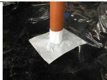
Typical pipe detail to core area 1.
