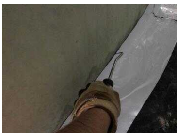
Testing along the lift shaft detail.
