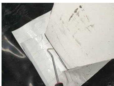
Stanchion detail testing
