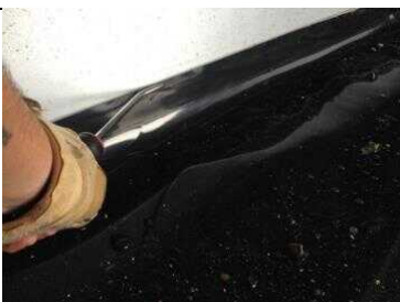
Testing along there perimeter cladding rail.
