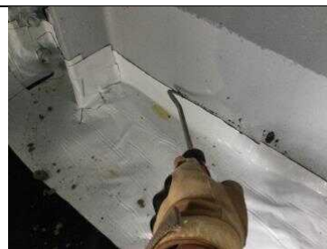
Testing to the stanchion detail within Core Area 1.
