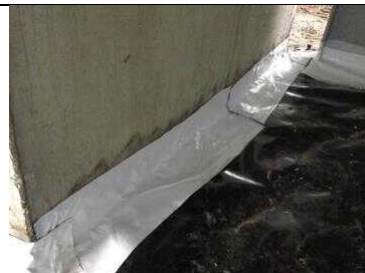
Retro detailing to lift shaft to core area 1.
