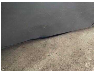
Compact substrate visible for inspection
