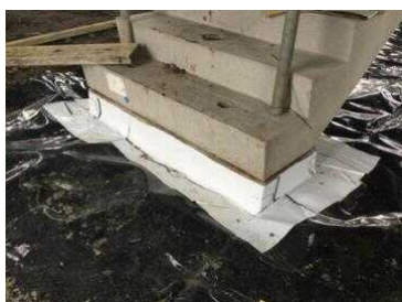
Stairwell base detailing to core area 2.
