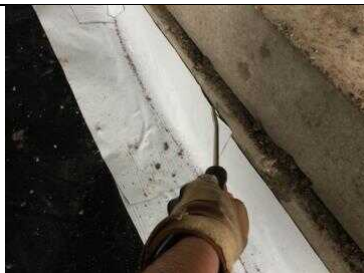
Testing to the stairwell base detail.
