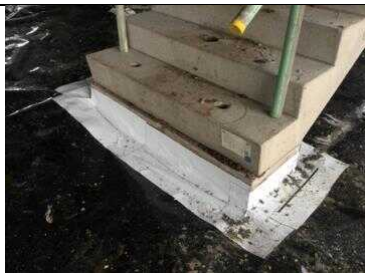
Stairwell base detailing to core area 1.
