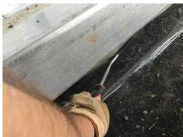
Testing to the perimeter cladding rail detail.
