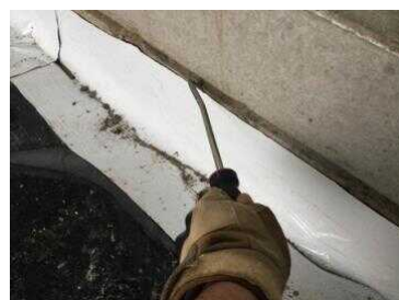
Testing along the stairwell base detail.
