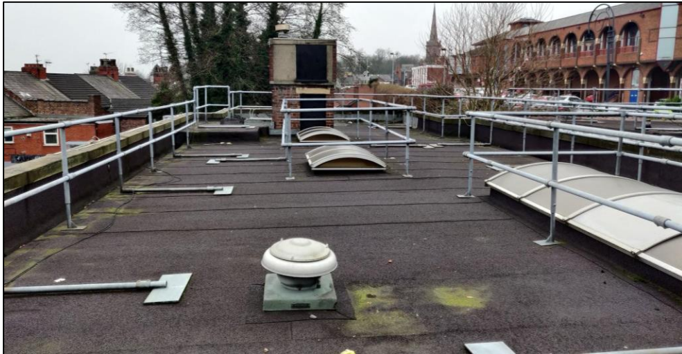
Photograph 6 showing the roof of Aspinall House
