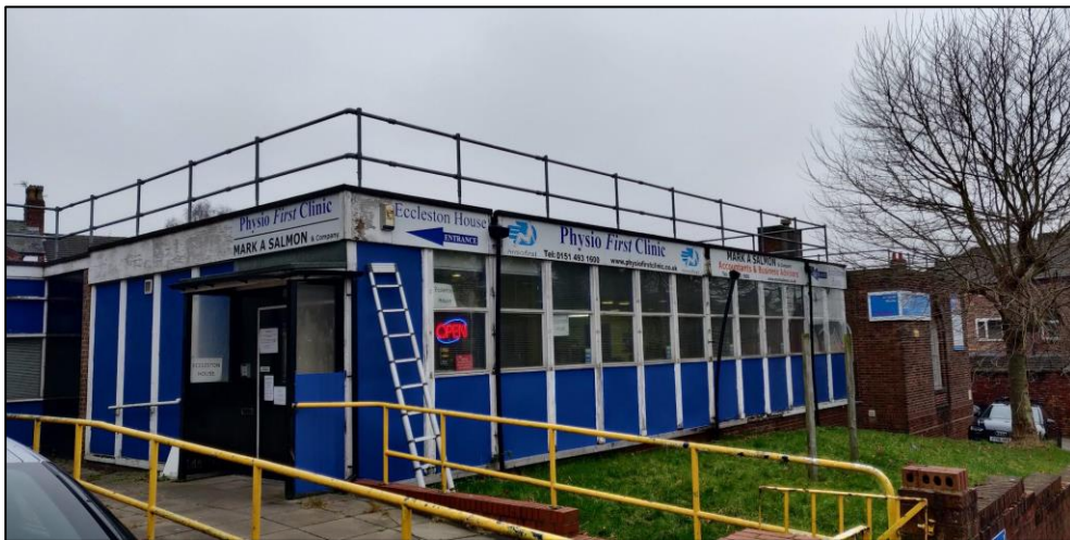
Photograph 1 showing the front elevation of the building
