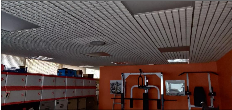
Photograph 4 showing an internal room at Eccleston House
