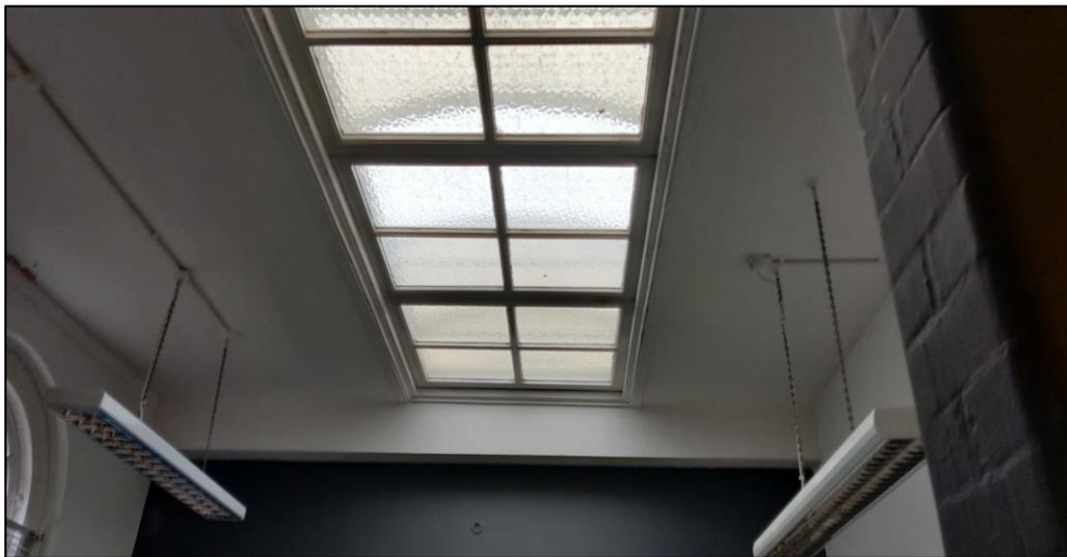
Photograph 7 showing part of the interior of Aspinall House
