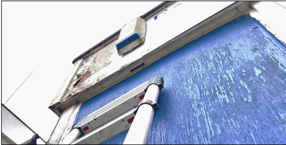
Photograph 2 showing the side elevation
