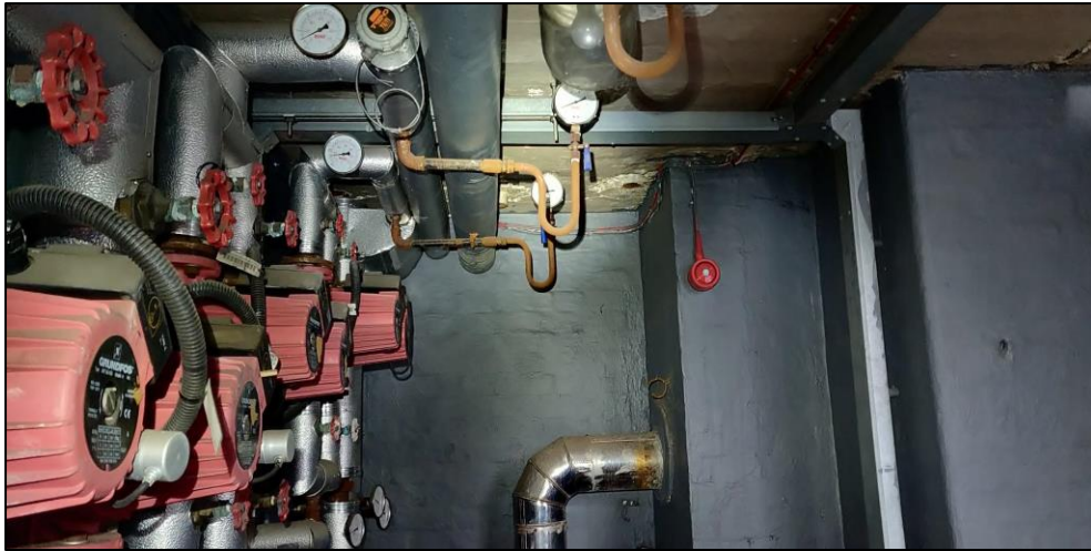
Photograph 8 showing the interior of the boiler room
