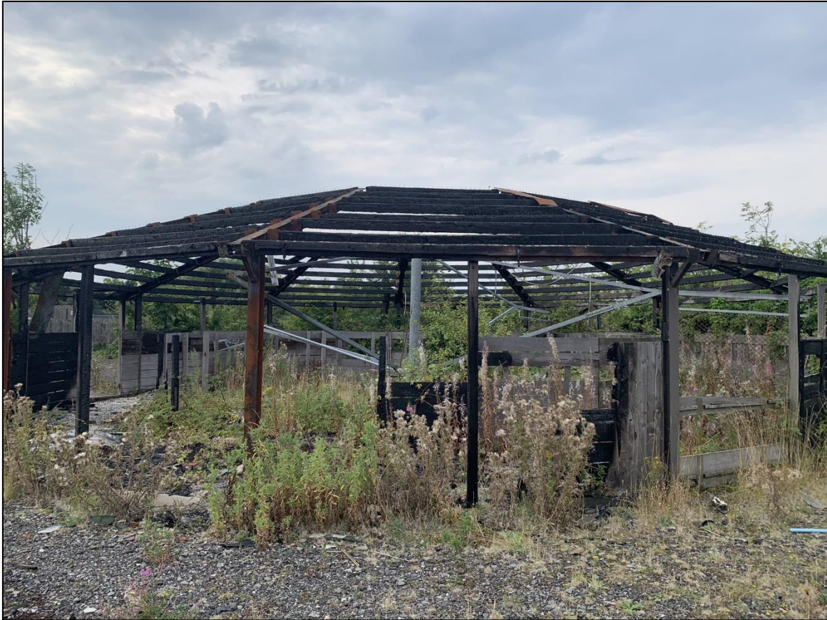
Plate 9 – Further angle of Building B2
