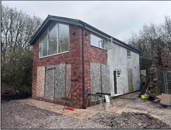
Figure 21: Building B1, viewed from the south.
