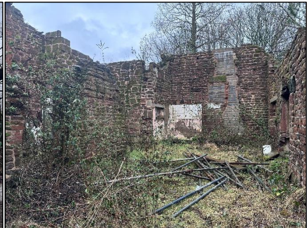
Figure 24: The interior of building B2.
