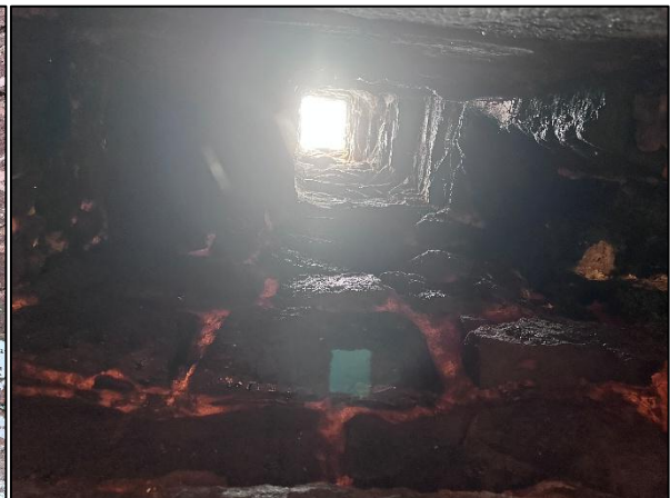
Figure 28: The chimney flue.
