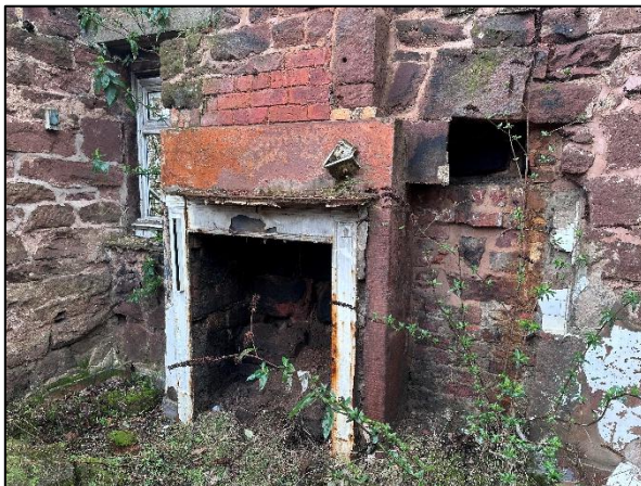
Figure 27: The old fireplace present inside the building.
