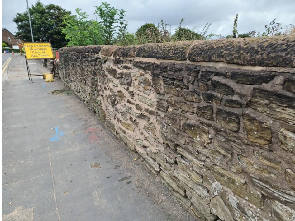
Image 1 - Sign of restoration work at the wall along Windy Arbor Road facing north
