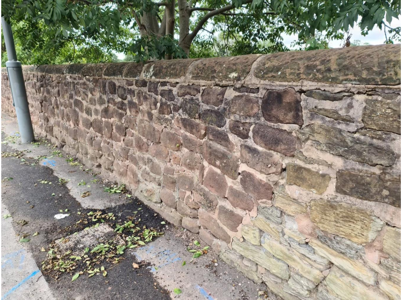
Image 3 - The two walls joining on Lickers Lane facing west
