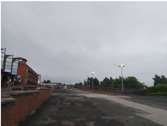
Main upper car park to the south of shopping centre (note lighting columns)
