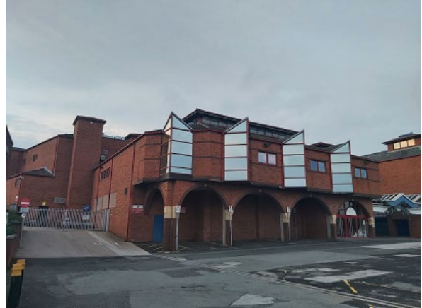
South Western aspect of Prescott Shopping Centre
