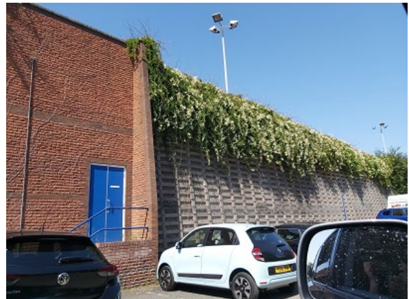
Lower car park and ornamental planting over retaining wall to south.
