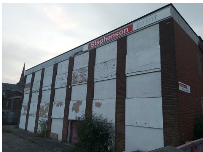
Disused Stephenson Print building to the west of the main shopping centre.
