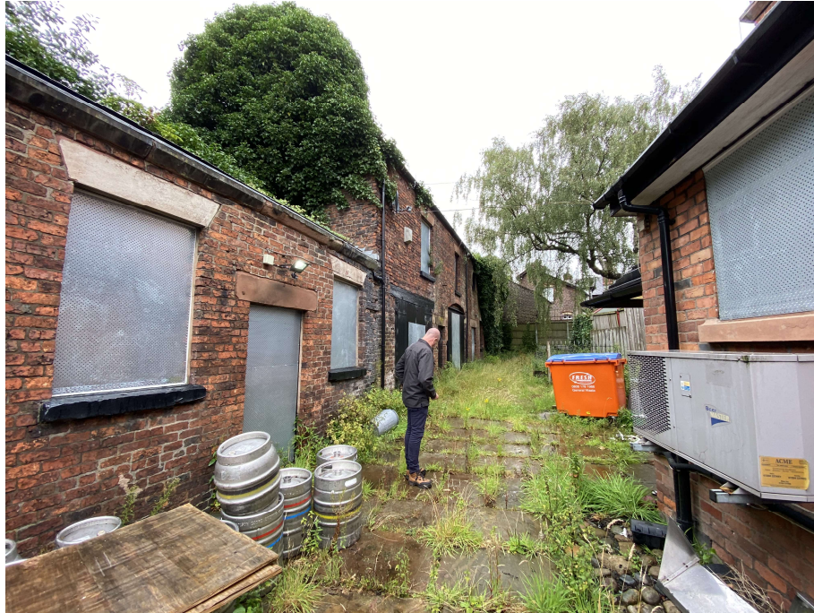
Plate 5 – Rear stable yard area with cellar colling units to the north elevation of the Clock Face to right of image.
