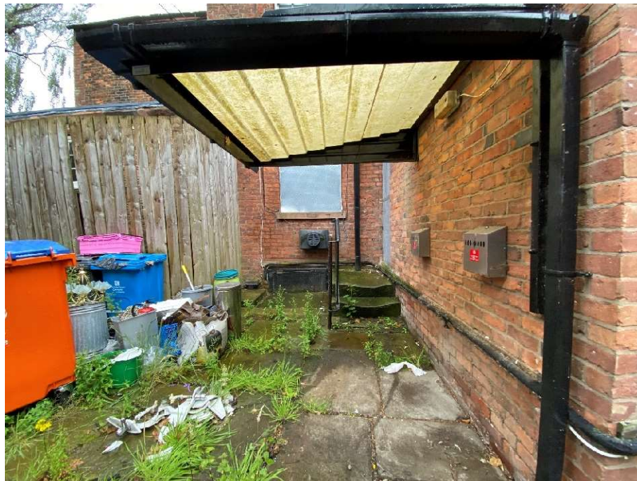
Plate 6 – Canopy shelter to the east elevation of the WC block of the Clock Face which is to be removed.
