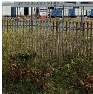
Boundary Treatment Existing metal palisade fence
