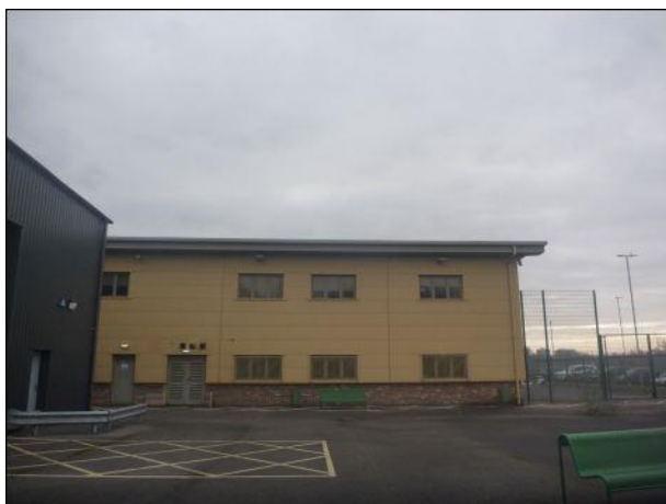
Photo 65: Building 4, western elevation, southern end
