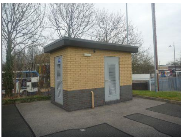
Photo 63: Building 3, southern and western elevations
