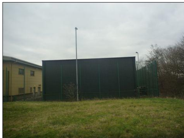
Photo 68: Building 5, northern elevation
