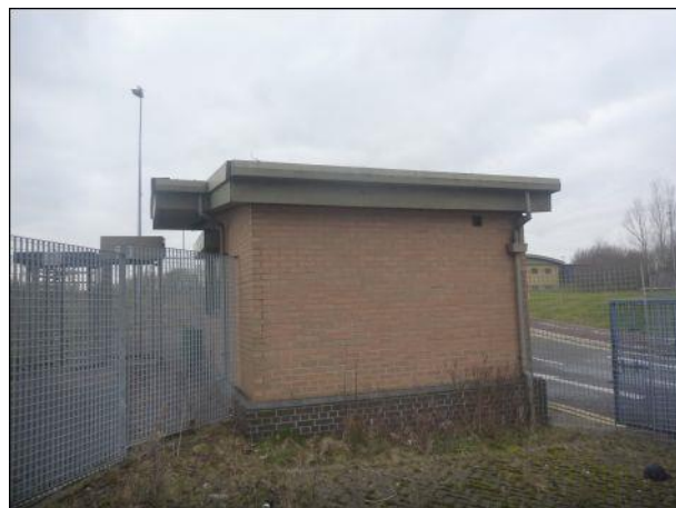
Photo 62: Building 2, northern elevation
