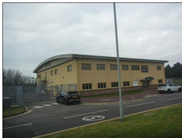
Photo 66: Building 4, southern and eastern elevations
