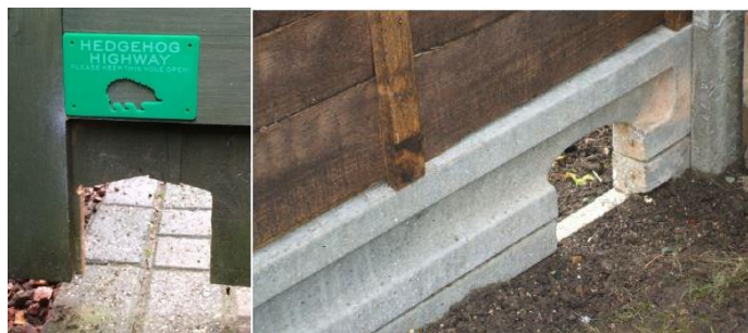
Insert 6: Showing wildlife access gap within fencing
