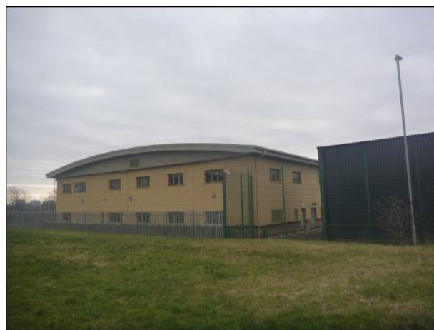
Photo 64: Building 4, northern and western elevations
