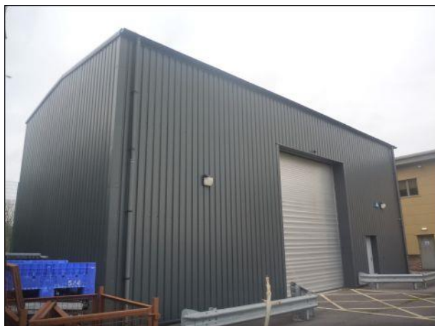
Photo 67: Building 5, western and southern elevations
