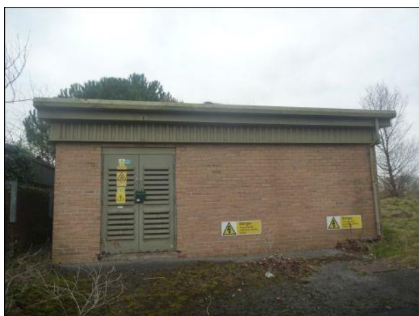
Photo 59: Building 1, northern elevation
