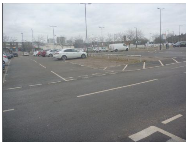
Photo 58: Hard standing within the car park area.
