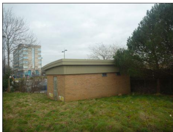
Photo 60: Building 1, western and southern elevations
