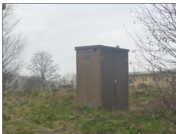
Photo 70: Structure 2, a small brick plant housing
