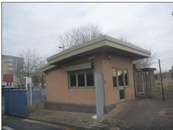
Photo 61: Building 2, western and southern elevations
