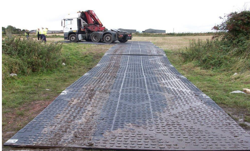
FIGURE 2: EXAMPLE OF GROUND PROTECTION MATS, IMAGE COURTESY MABEYHIRE.CO.UK
