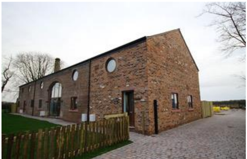
Photo B2. Existing Buildings
