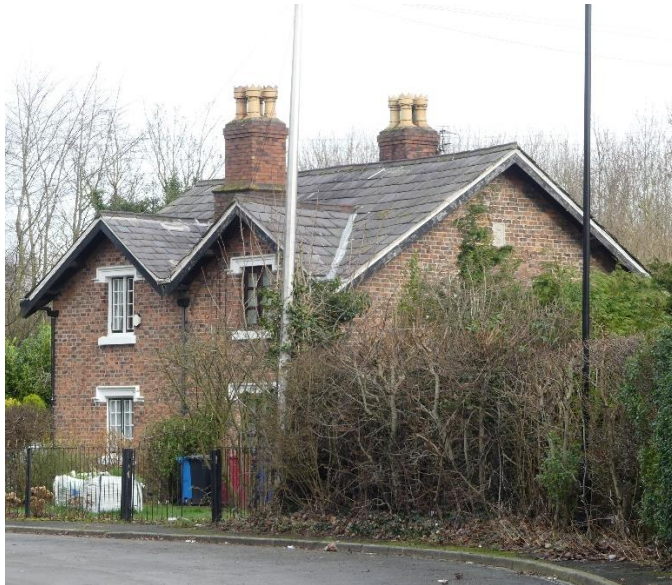
Figure 4.8: Nos. 1 and 2 Ingoe Lane
