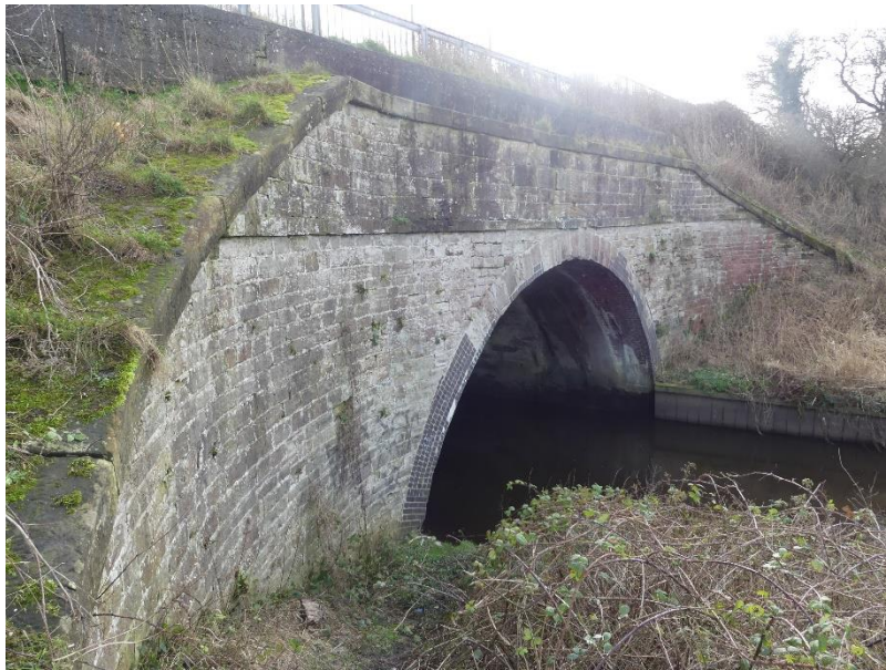
Figure 4.12: The northern elevation of The Culvert
