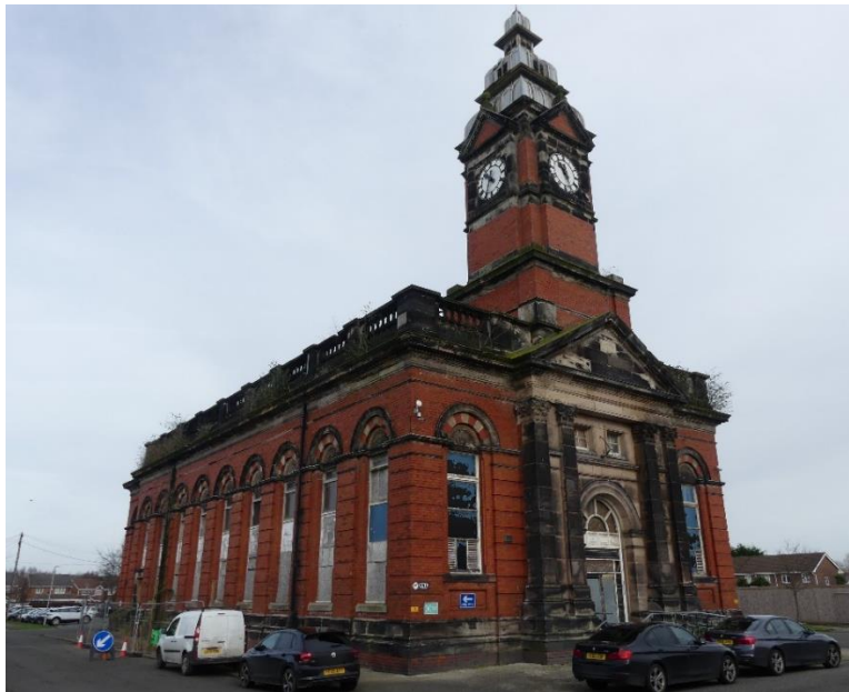
Figure 4.2: The portico and tower of the Dining Room
