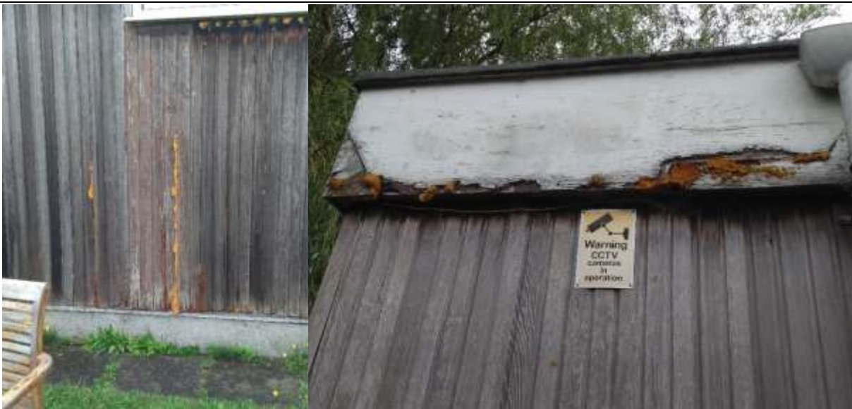
Photo 12: Building 2 (2020) showing the expanding foam on the south eastern and north western elevations.
