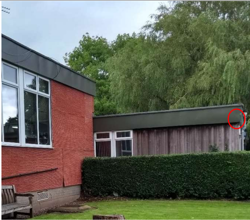
Photo 13: Building 2 showing the roost location on the south western elevation.
