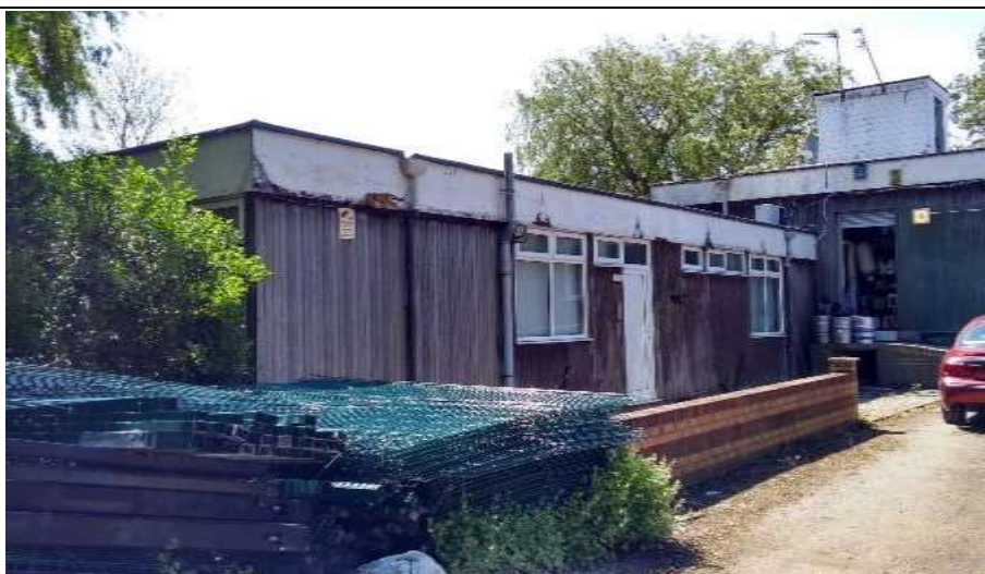
Photo 5: North-eastern elevation of Building 2 (foreground) and south-eastern end of Building 1 (background).
