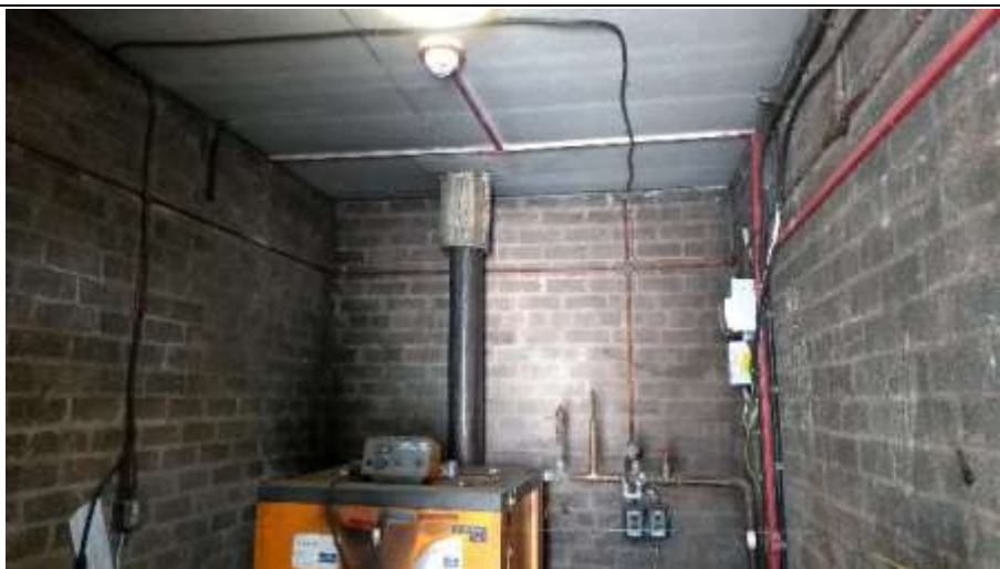
Photo 9: Internal room within Building 3.
