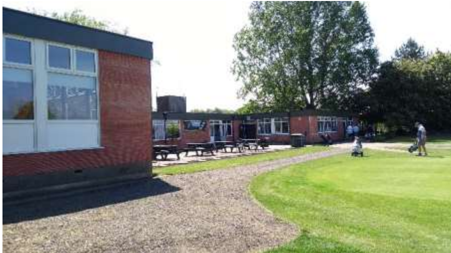
Photo 3: North-eastern elevation of Building 1.
