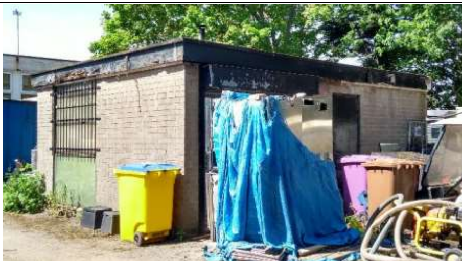
Photo 7: South-western and south-eastern elevations of Building 3.
