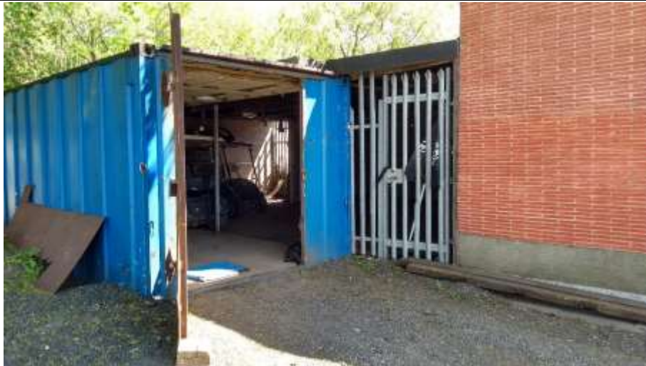
Photo 10: View from north of Building 4.
