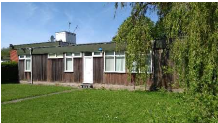
Photo 4: South-western elevation of Building 2.
