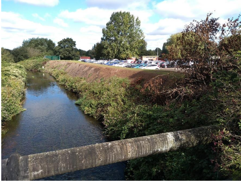
Photograph 3: Area of bank adjacent to the car park affected by works (September 2020).
