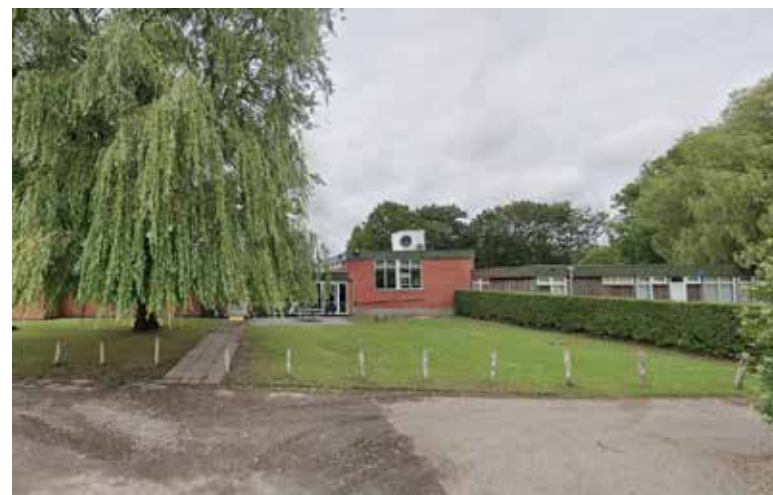
Figure 8. Existing golf club front elevation
