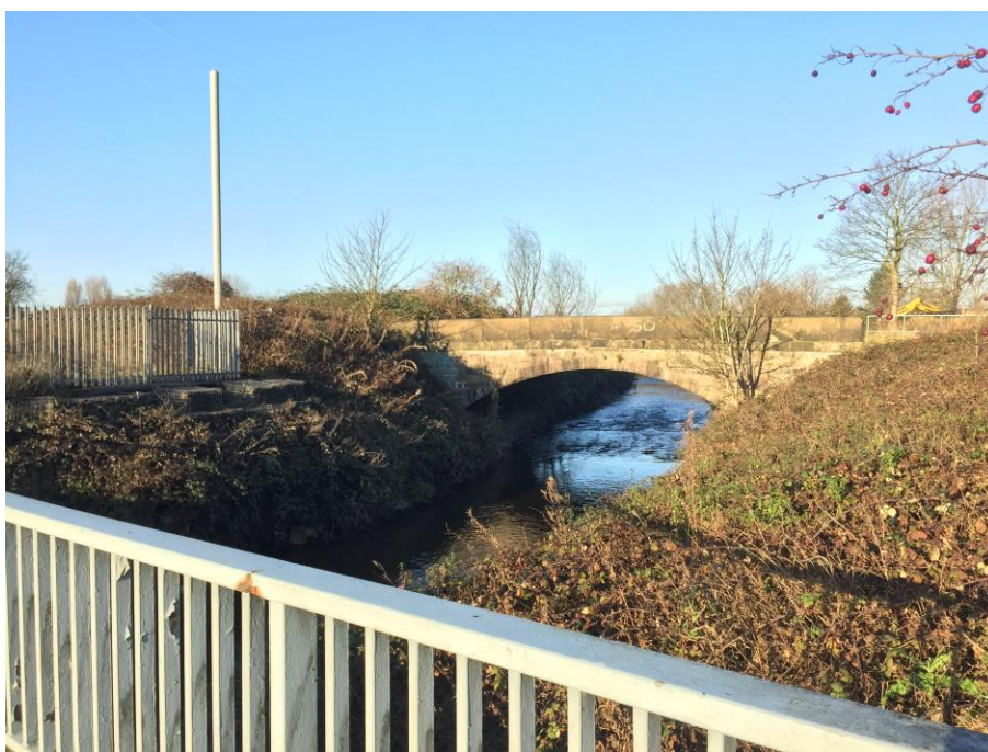
Figure 8: View north-west showing Alder's Bridge
