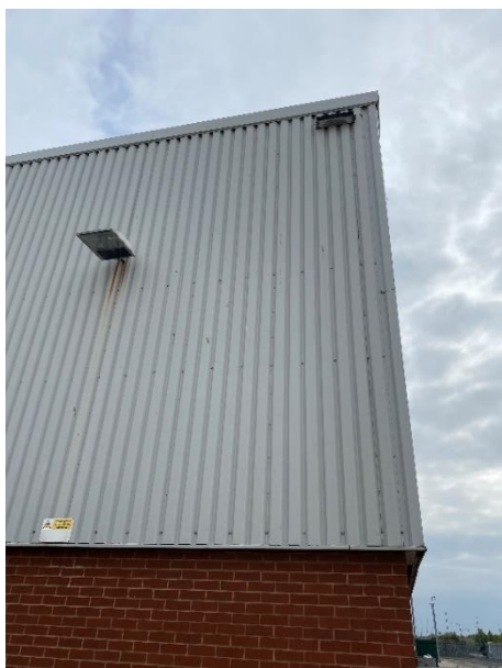
Photograph 1 – Southern elevation of Building 1 (B1)
