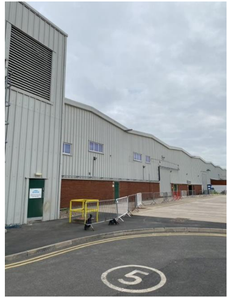
Photograph 6 – Southern elevation of B2
