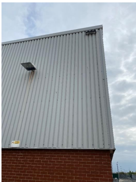
Photograph 1 – Southern elevation of Building 1 (B1)
