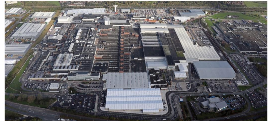
Figure 3 – Jaguar Land Rover Halewood with the previous temporary tent to the south
