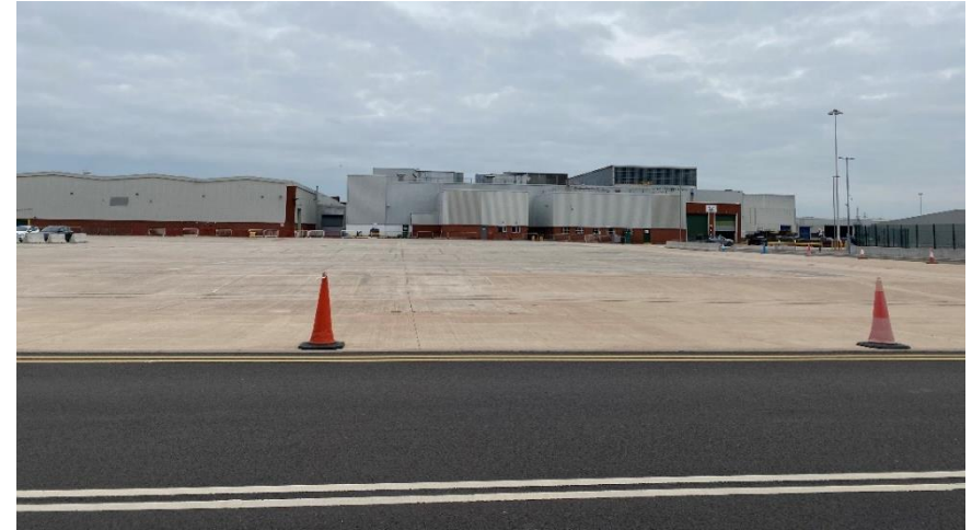
Figure 2 - Existing hardstanding following removal of temporary tents
