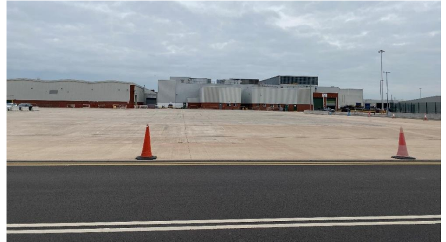
Figure 2 - Existing hardstanding following removal of temporary tents
