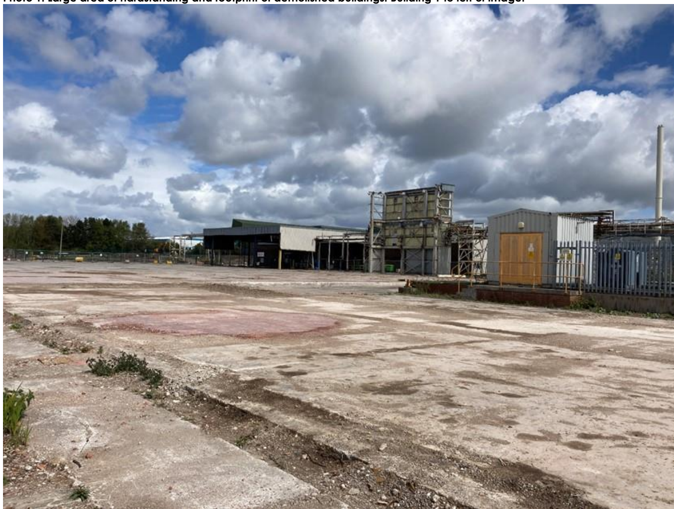
Photo 1: Large area of hardstanding and footprint of demolished buildings. Building 1 to left of image.
