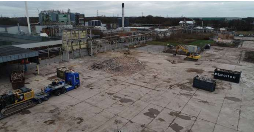
3. View of Site 3 looking south west during demolition
