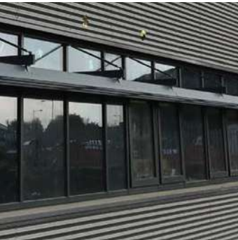
Ribbon Windows with integrated Brise Solail.
