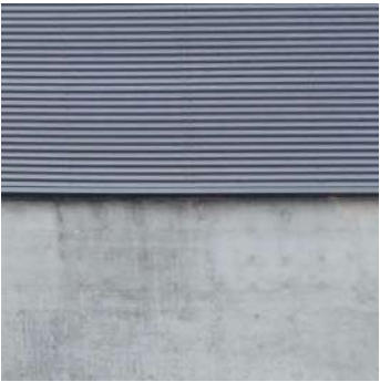
Precast concrete wall
