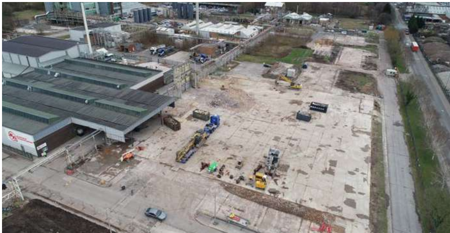
4. Boundary along Acornfield Road looking North, at now demolished office building
