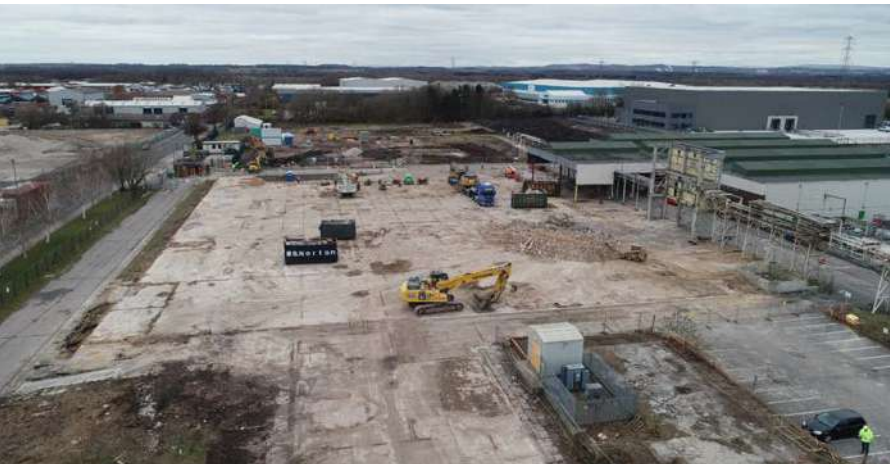
5. View north east from inside site 3
