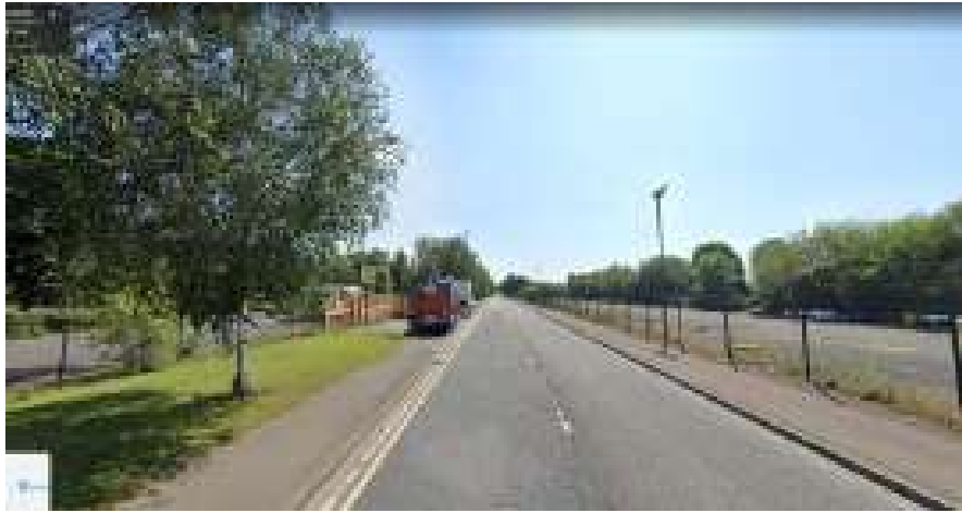
1. View south along Acornfield Road
