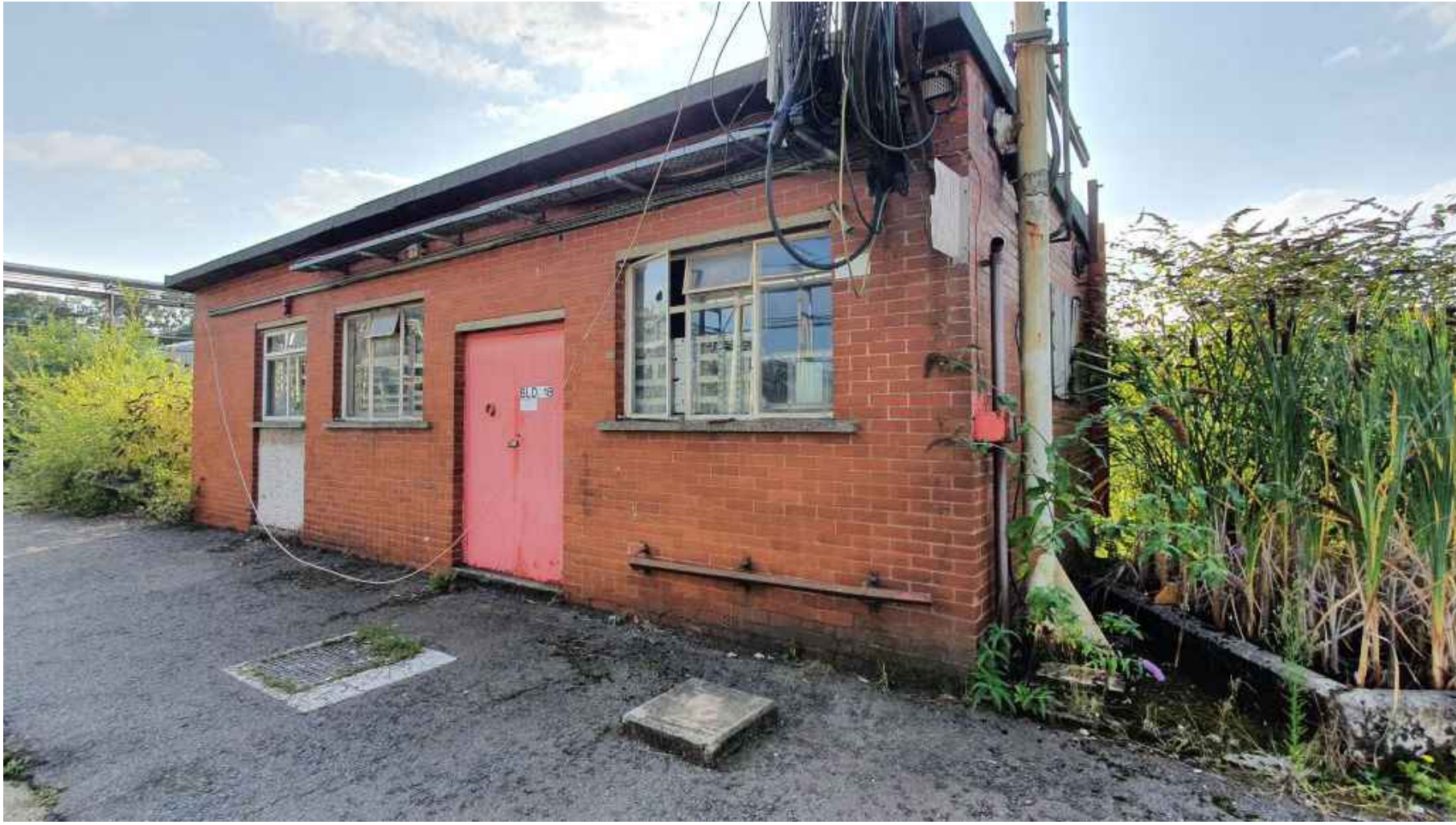
02 Building 18 Existing - Photograph of North/ East Elevation 1:2000 @ A1
