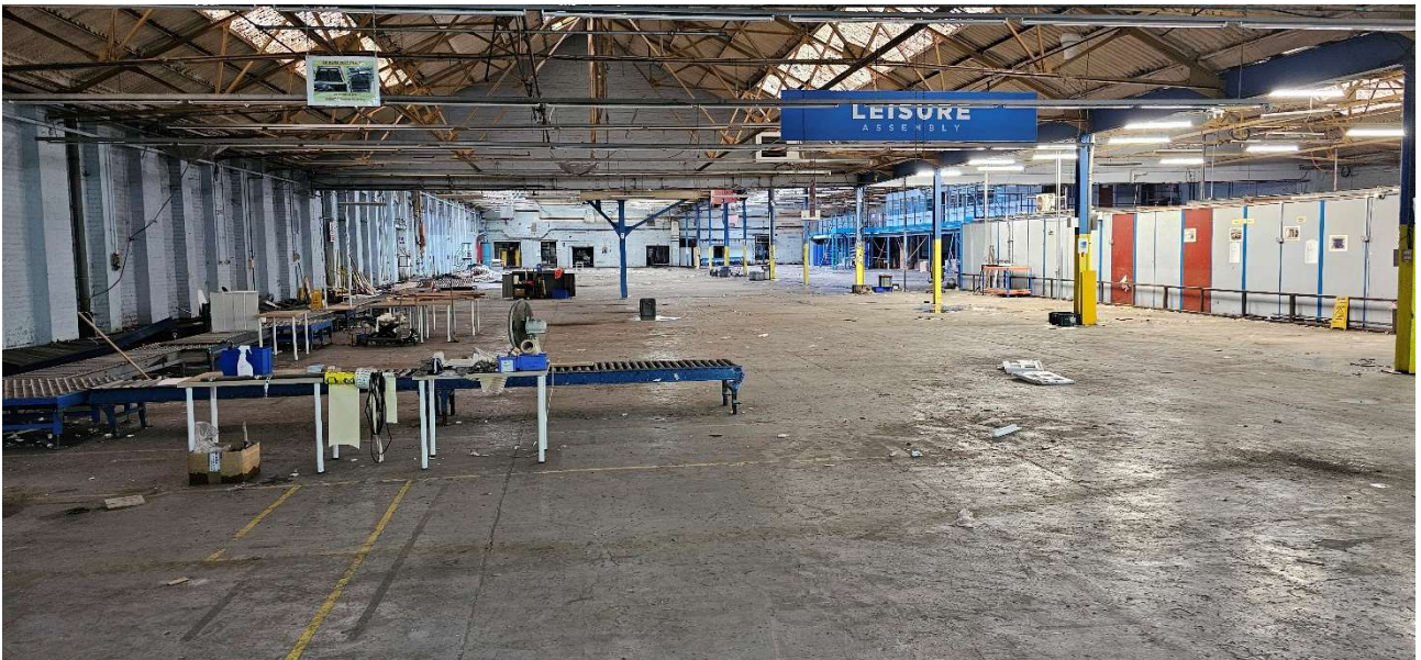
Image1E(2) – Interior of Building 1E looking east
