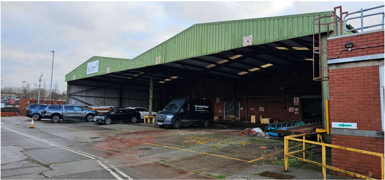
Image 1B(1) – Building 1B viewed from the south west
