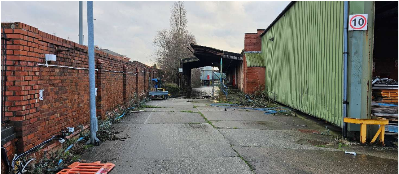
Image 1D(1) – Building 1D (canopy) viewed from the west
