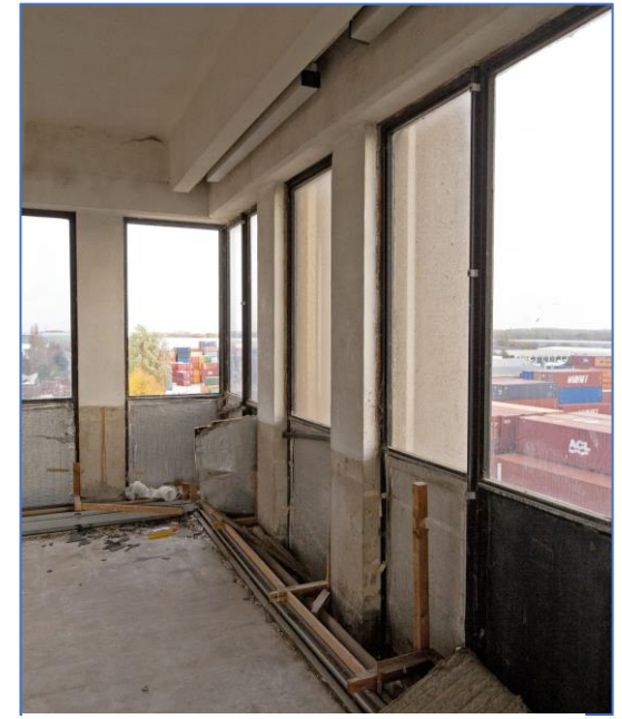
Figure 6 – Photo of Inside of Windows
