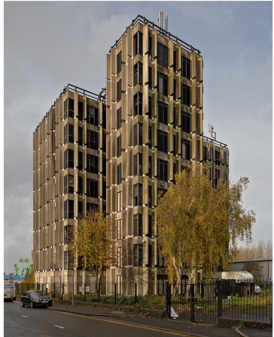
Figure 2 – Photo of existing building from South East – November 2023
