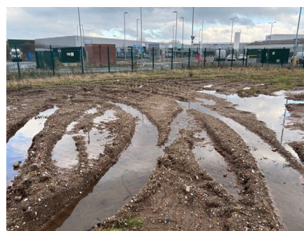
Surface water ponding in the south-east.
