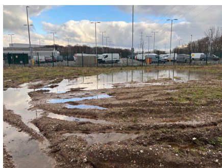
Surface water ponding in the east of site.
