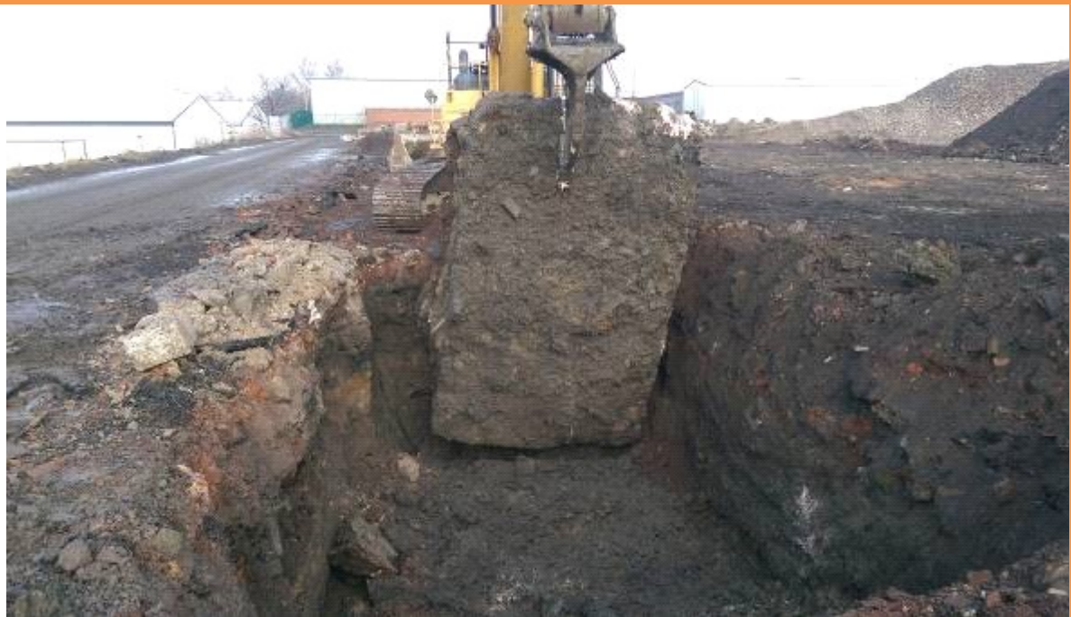
PLATE 11 – SMALL RELIC FOUNDATIONS BEING REMOVED PRIOR TO TURNOVER
