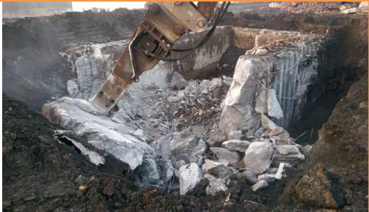
PLATE 8 – LARGE UST BEING BROKEN TO AID IN THE REMOVAL OF THE TANK
