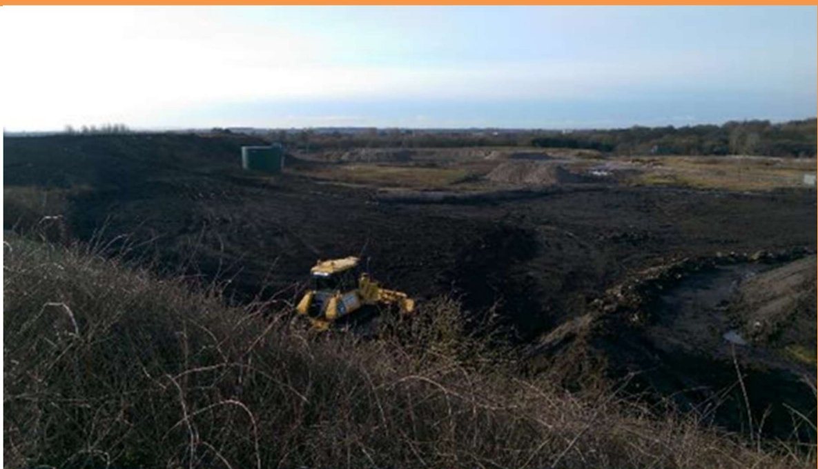
PLATE 14 – VIEW WEST OF LOWER PARCEL C WITH TURNOVER OF >1.50BGL COMPLETED TO NATURAL STRATUM
