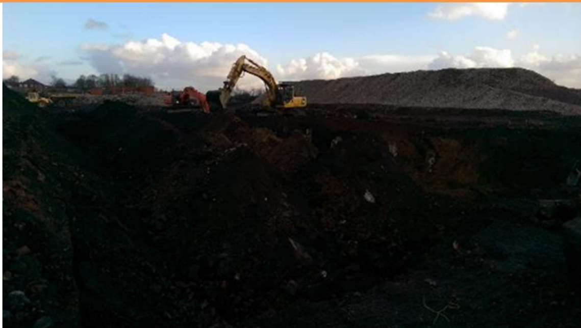
PLATE 6 – TURNOVER AND REMOVAL OF RELIC STRUCTURES
