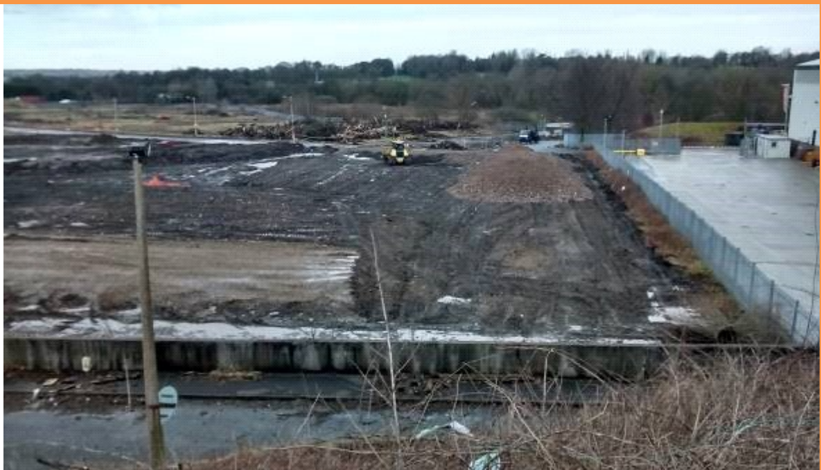
PLATE 16 – NORTHERN LOWER AREA OF PARCEL C WITH COMPOUND BEING CONSTRUCTED
