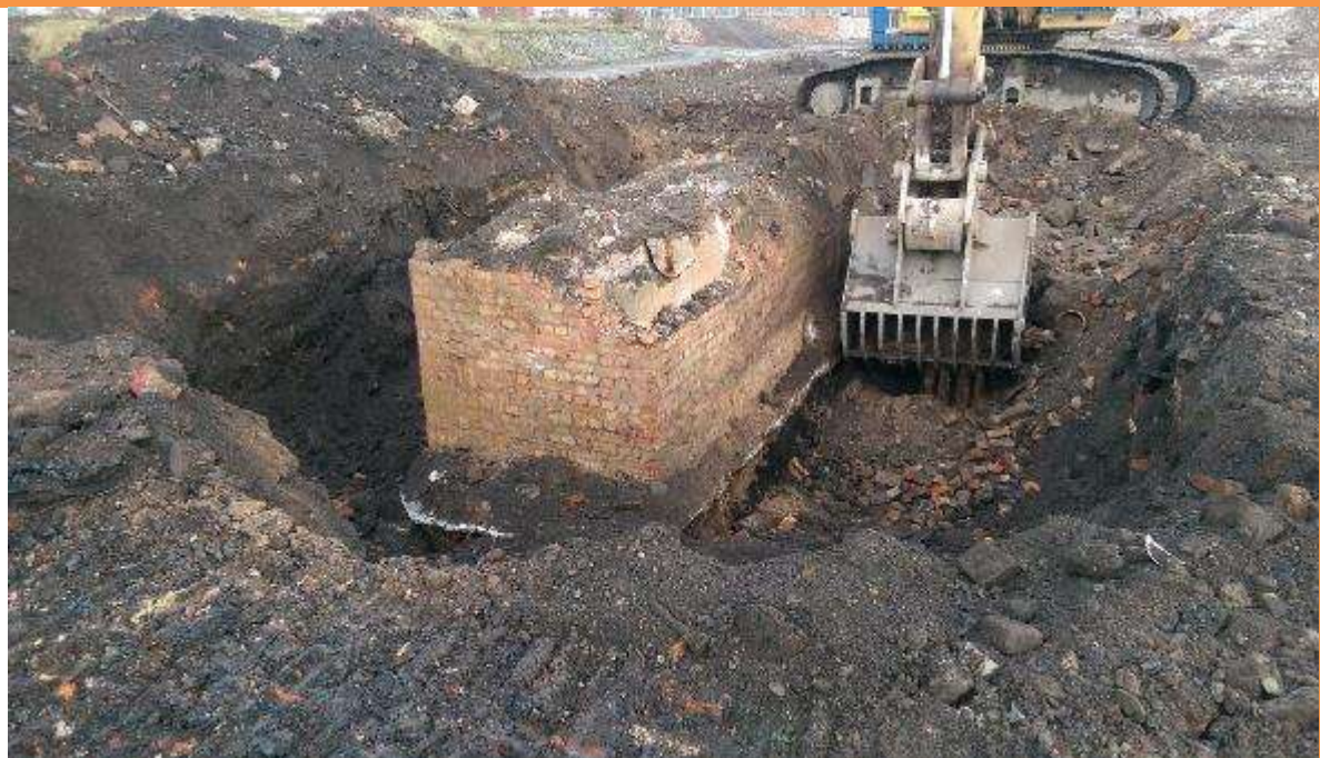
PLATE 4 - TURNOVER OF REMOVAL OF RELIC STRUCTURES IN UPPER EAST OF PARCEL C
