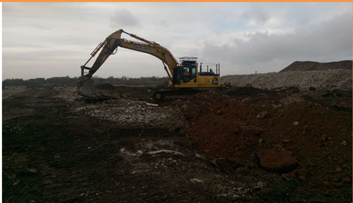
PLATE 9 - LAST REMAINING AREA OF TURNOVER WITHIN UPPER PORTION OF PARCEL C
