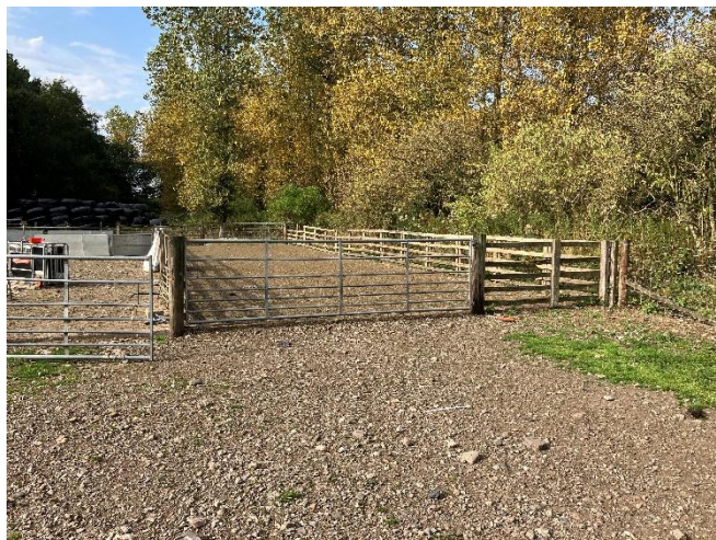
Fig. 3 – further general view (existing sheep pen).
