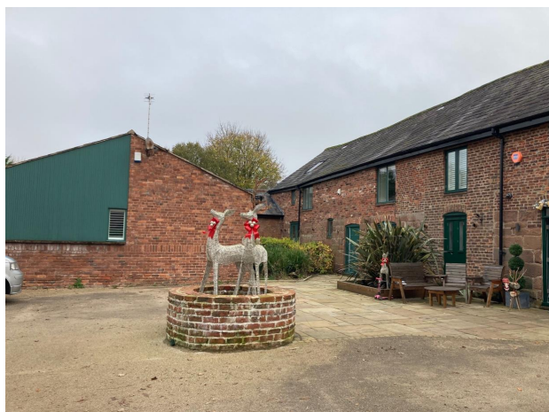
Fig.14 View into courtyard of Shippons 2 & 3
