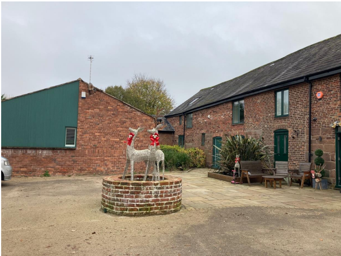
Fig.1 East elevation of Shippons 2 & 3 with South gable end of Shippon 1
