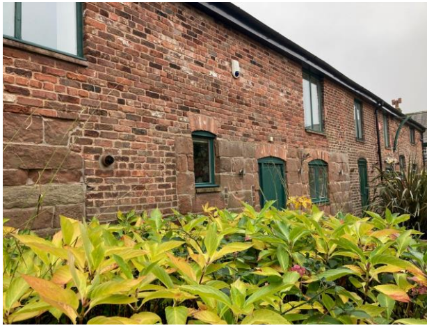
Fig.15 Elevation mixture of brick & sandstone block
