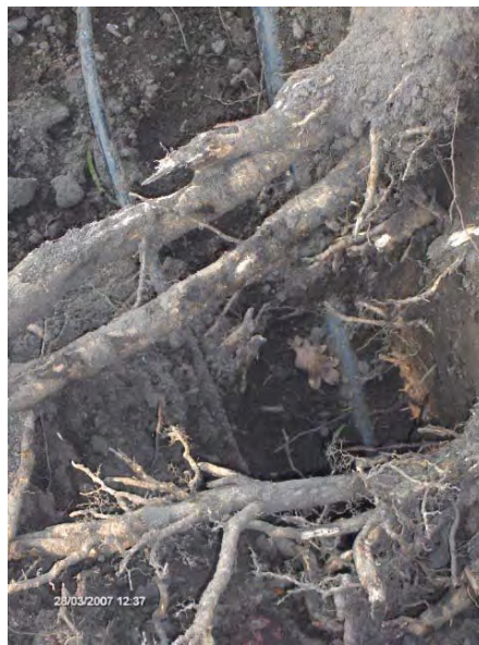
Typical root damage caused by excavation works
