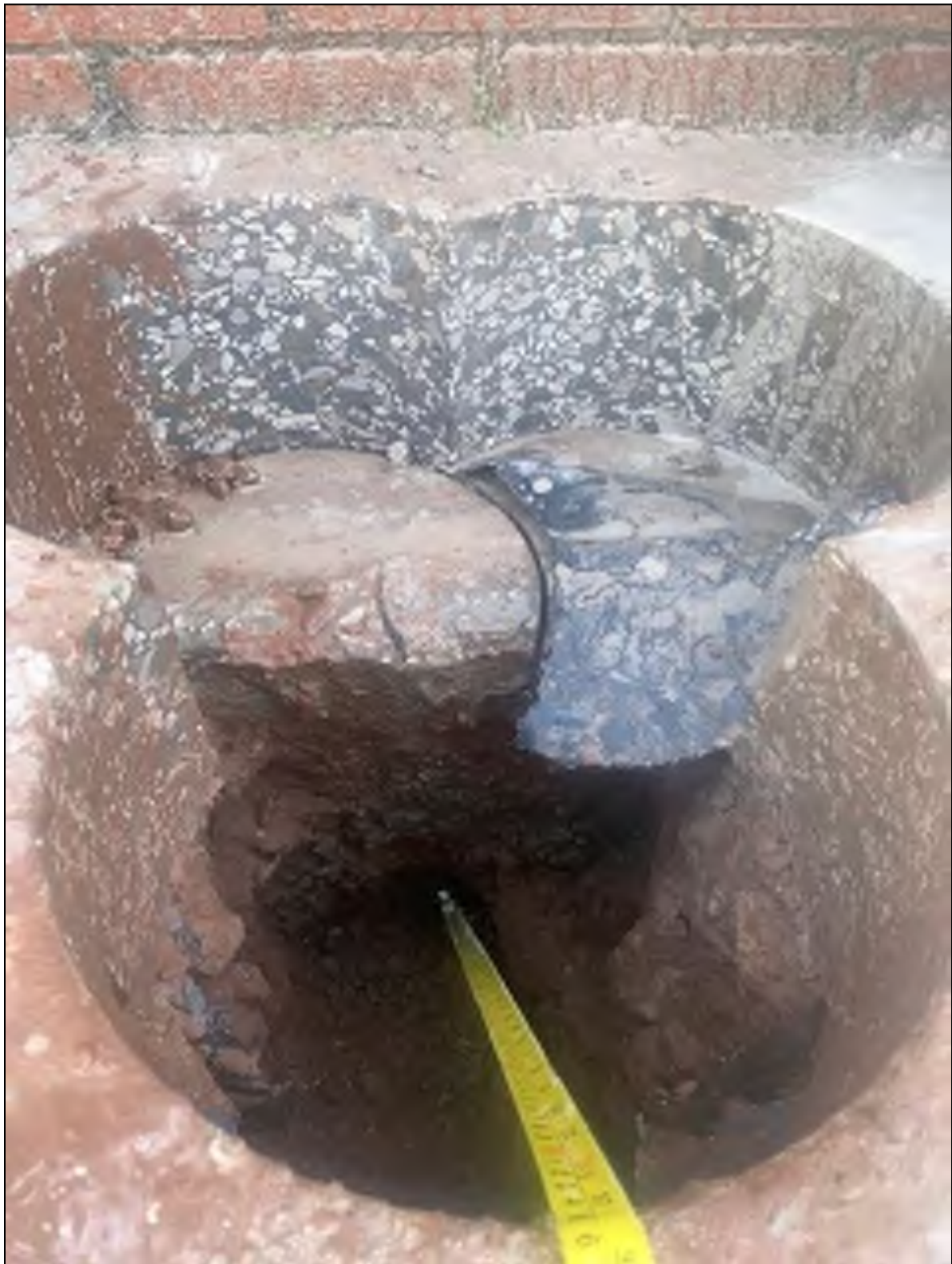
Photo Plate No. 18: Foundation pit 02 showing tapering strip footing foundation.
