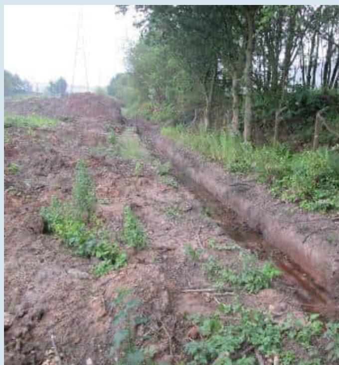
Photograph 10: Target Note 4, recently excavated section of dry ditch which links up with a natural watercourse running along southern Site boundary.
