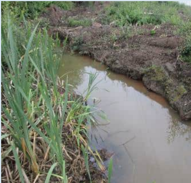
Photograph 7: Target Note 1, section of wet ditch which was recently been excavated, between the site of a dry pond and Briton Plantation woodland.
