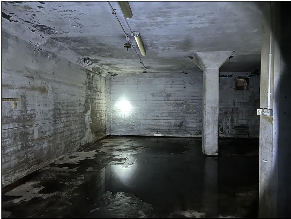
Plate 5 – Nature of the interior of the bunker
