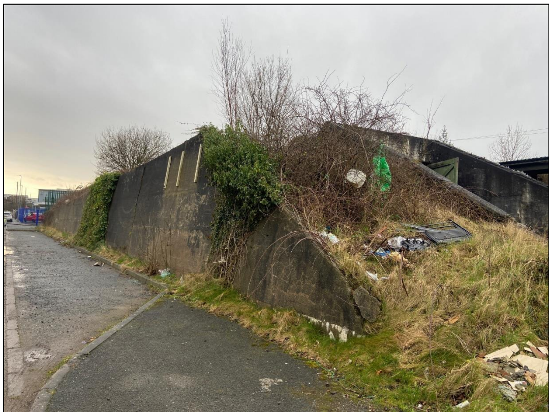
Plate 2 – Character of the bunker as viewed from Draw Well Road to the east
