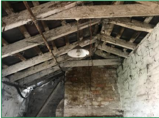
The interior of the middle section of the outbuilding
