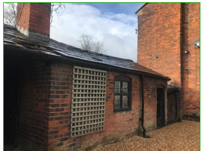
The northeast elevation of the outbuilding
