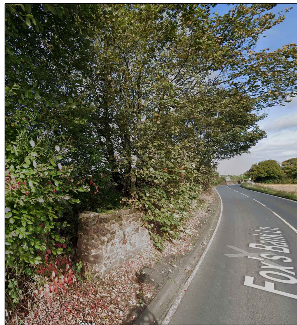
Google Street View Photographs of Low Level Wall - NTS
