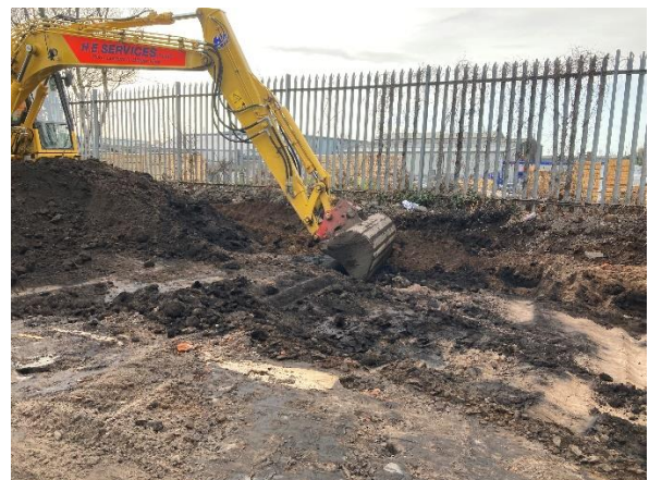
Plate 6 Excavating Peat in the North
