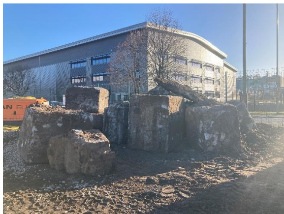
Plate 5 Oversize Removed from Reduced Level Dig
