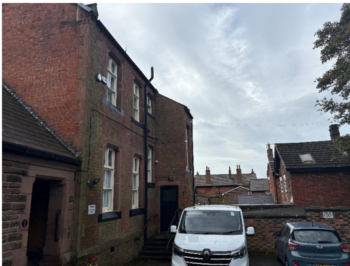
The Presbytery frontage looking west
