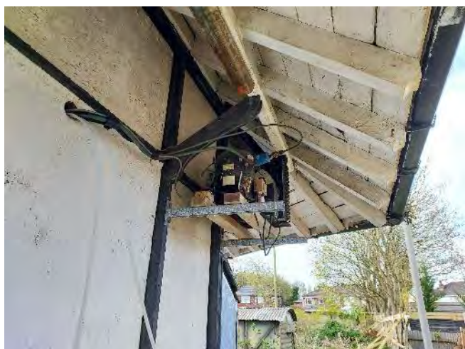
Figure 13 – Disused services within the former cricket club building, looking north-east.
