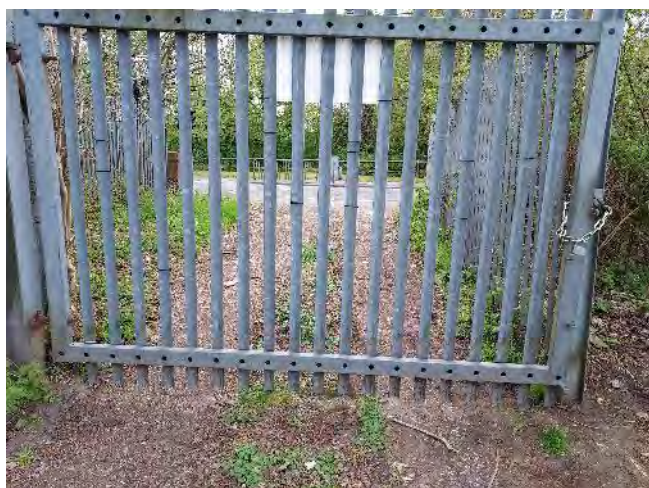
Figure 1 – Access gate to the site in the northern site section, looking north-east.
