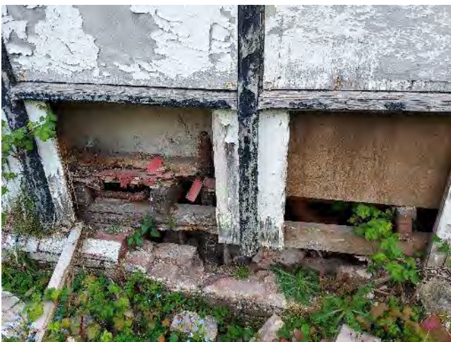
Figure 11 – Disused services into the cricket club building, looking north-east.
