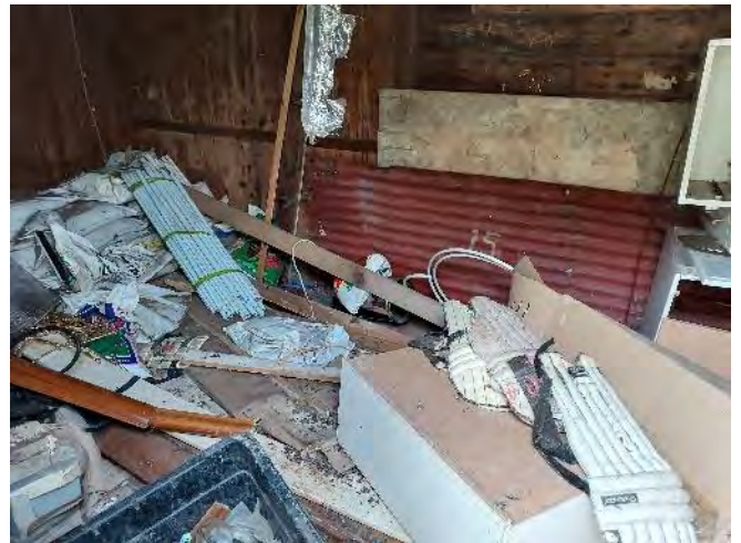
Figure 10 – The interior of the on-site shed, looking north.
