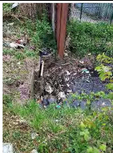
Figure 2 – The River Alt culvert along the northern site boundary, looking north.
