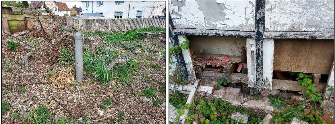
Figures 8 & 9: Evidence for a disused street light system (left) and on-site services into the buildings (right).
