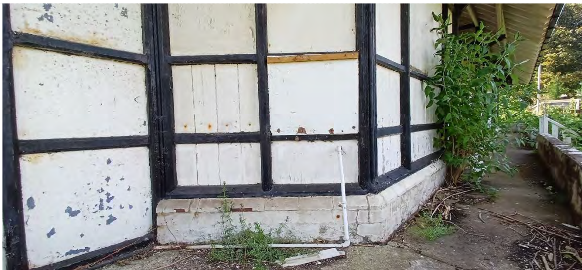
Figure 28 – Retaining wall to rear veranda
