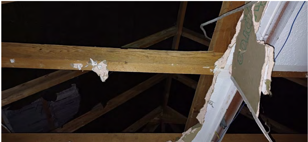
Figure 76 – Right toilet room
