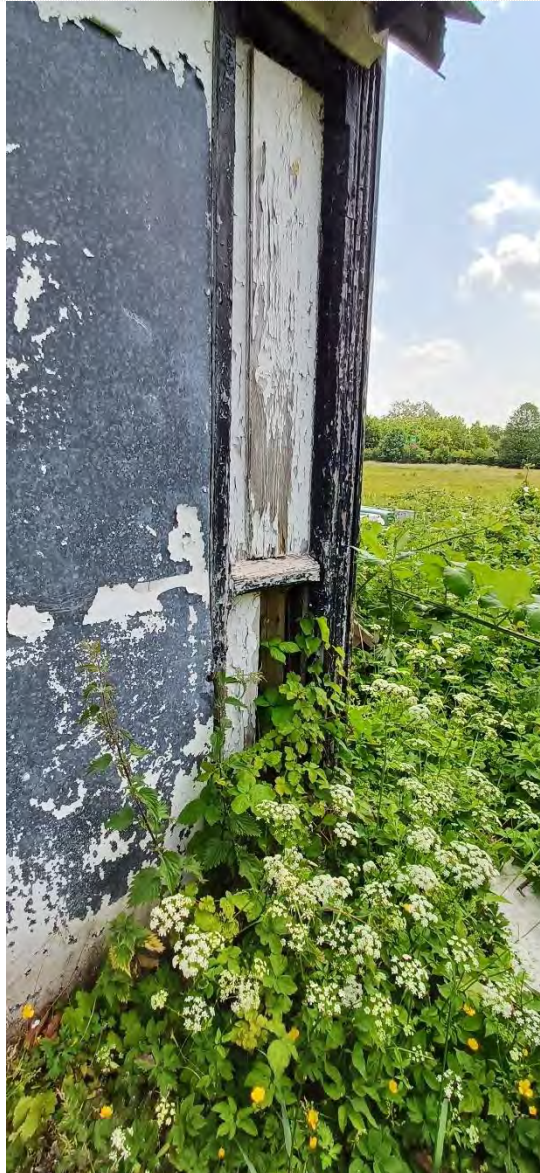
Figure 48 – Front left corner
