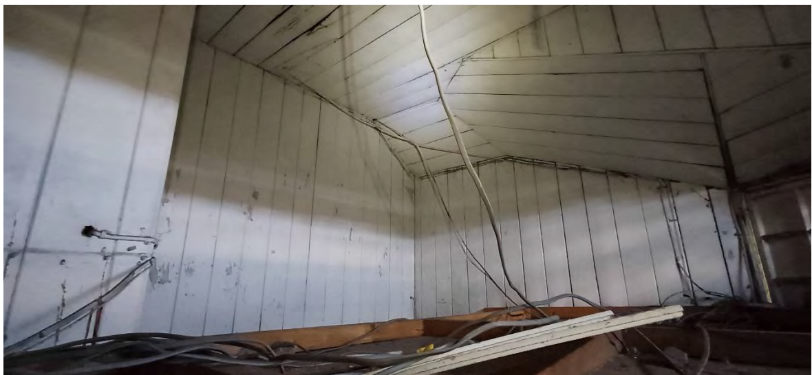
Figure 92 – Former window, rear wall to bar
