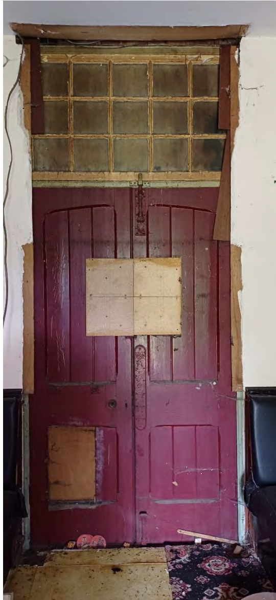
Figure 57 – Central doors, rear wall
