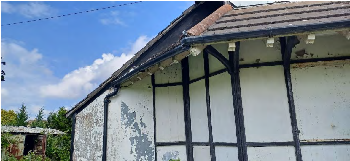
Figure 7 – Damaged brickwork/render to retaining wall
