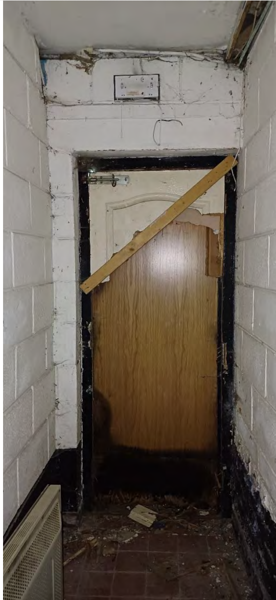
Figure 75 – Door to front wall
