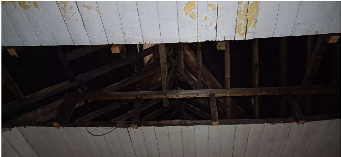
Figure 58 – Right hand room, main building
