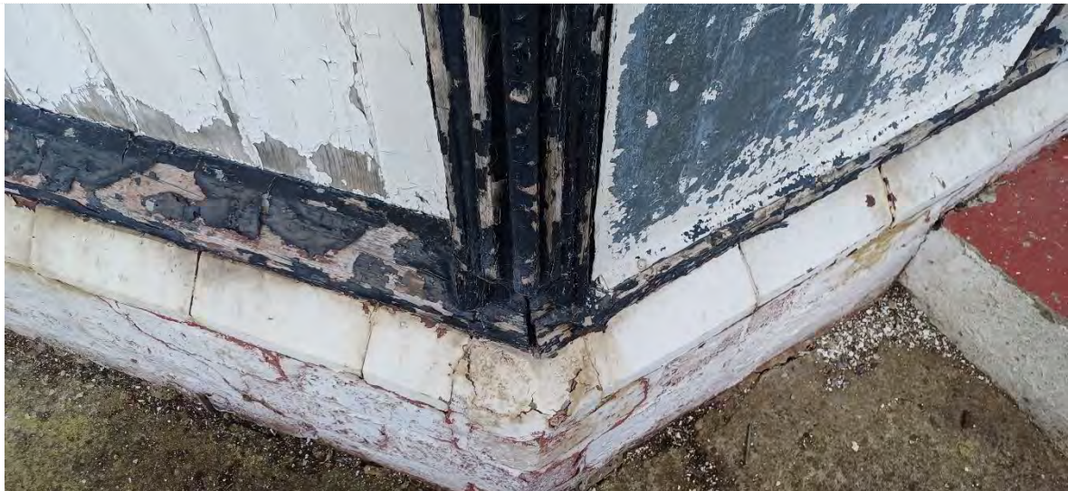
Figure 38 – Ply panelling adjacent to lathe panel
