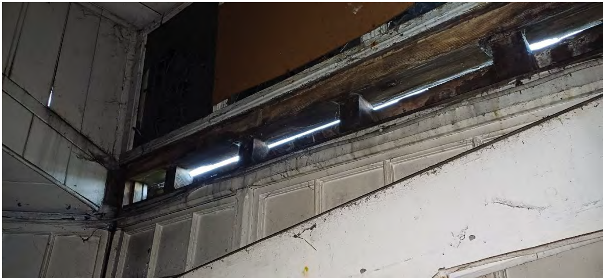
Figure 90 – Roof – right side of right room
