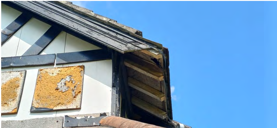
Figure 17 – Boarding to roof, left side of right dormer
