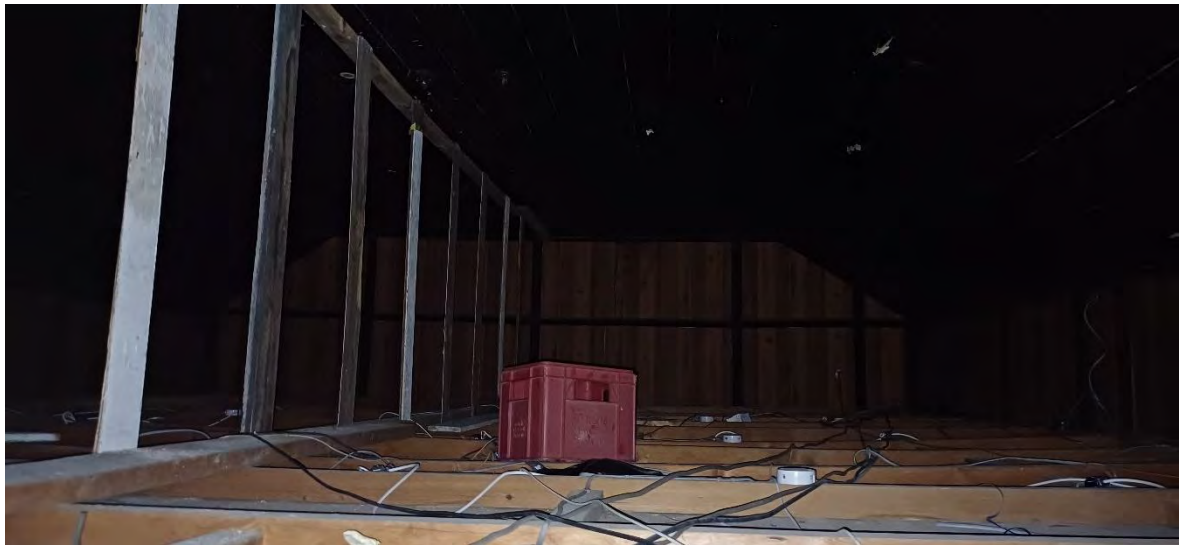
Figure 88 – Opening to left of kitchen
