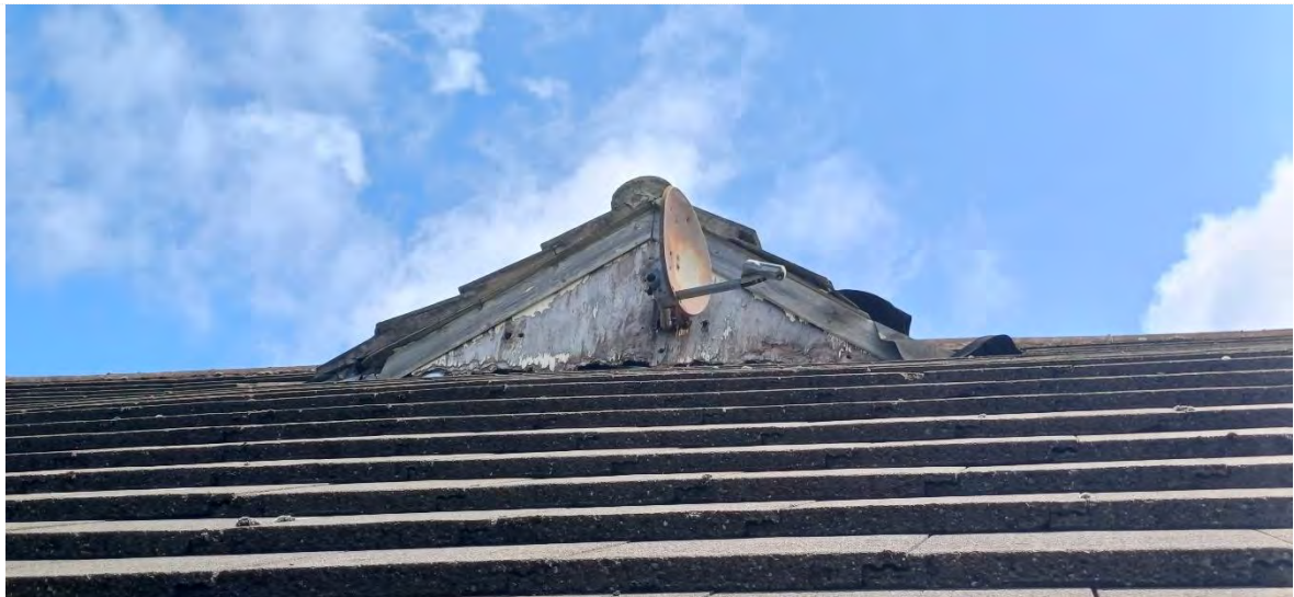
Figure 49 – Front left corner
