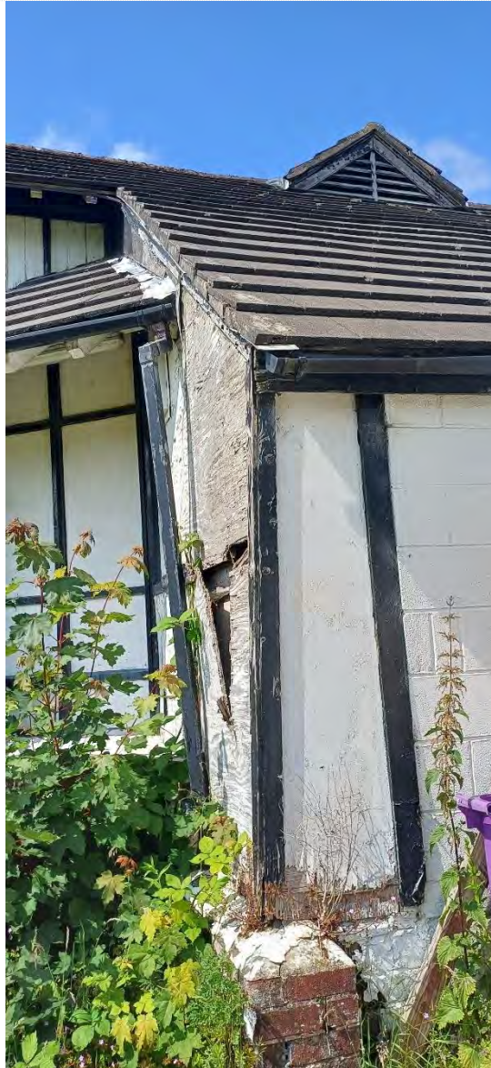
Figure 20 – Cladding & corner non-vertical
