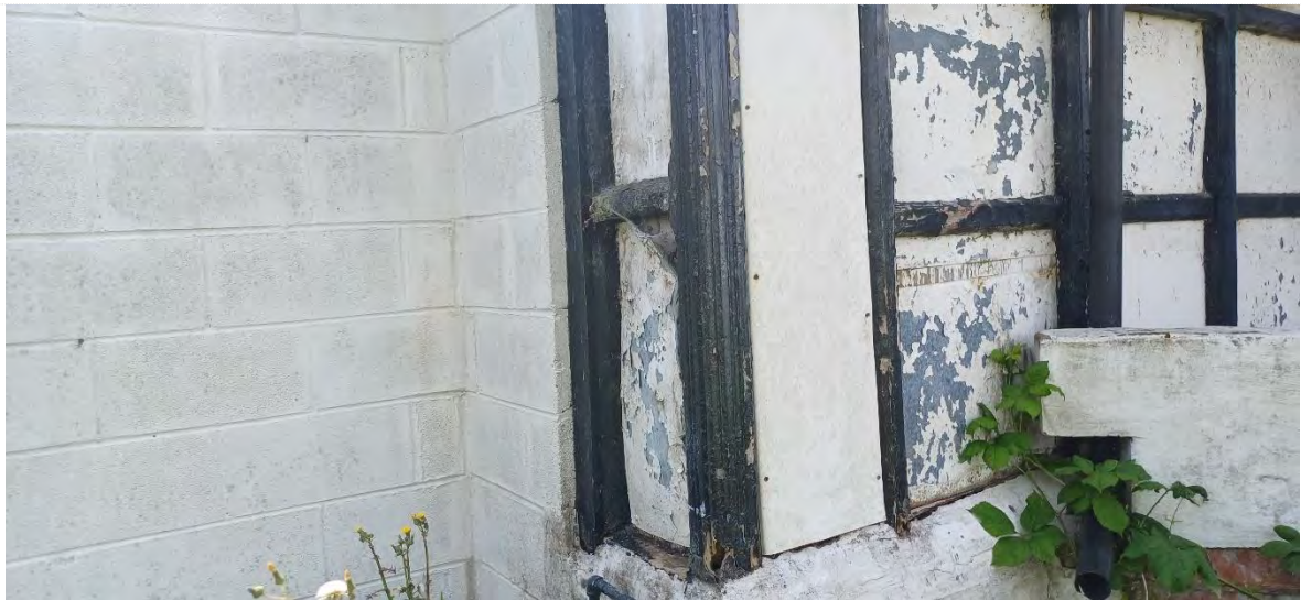
Figure 25 – Uneven ridge tiles, right side, rear
