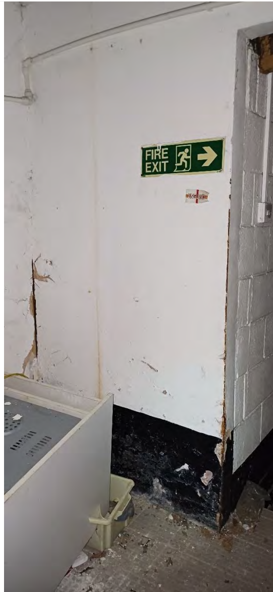
Figure 71 – Rear of right wall toilets
