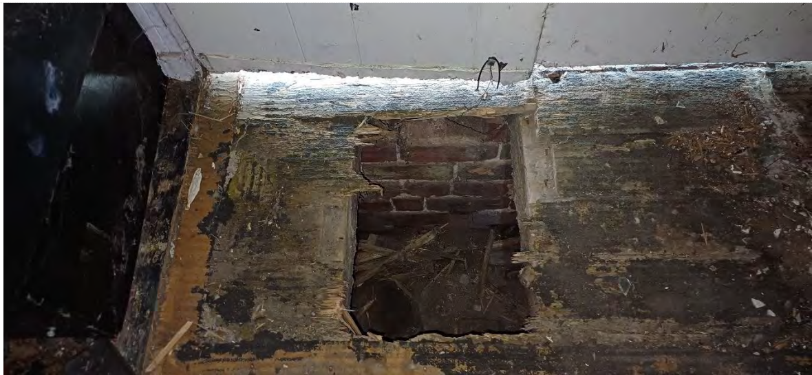
Figure 78 – Sleeper wall, right room
