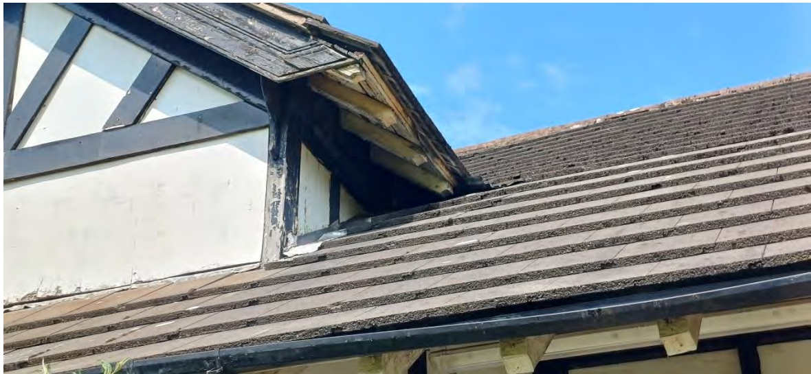
Figure 11 – Flashing detail, left dormer
