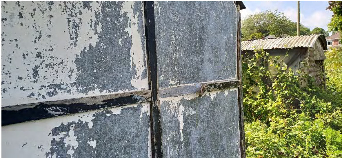
Figure 40 – Left end of rear elevation
