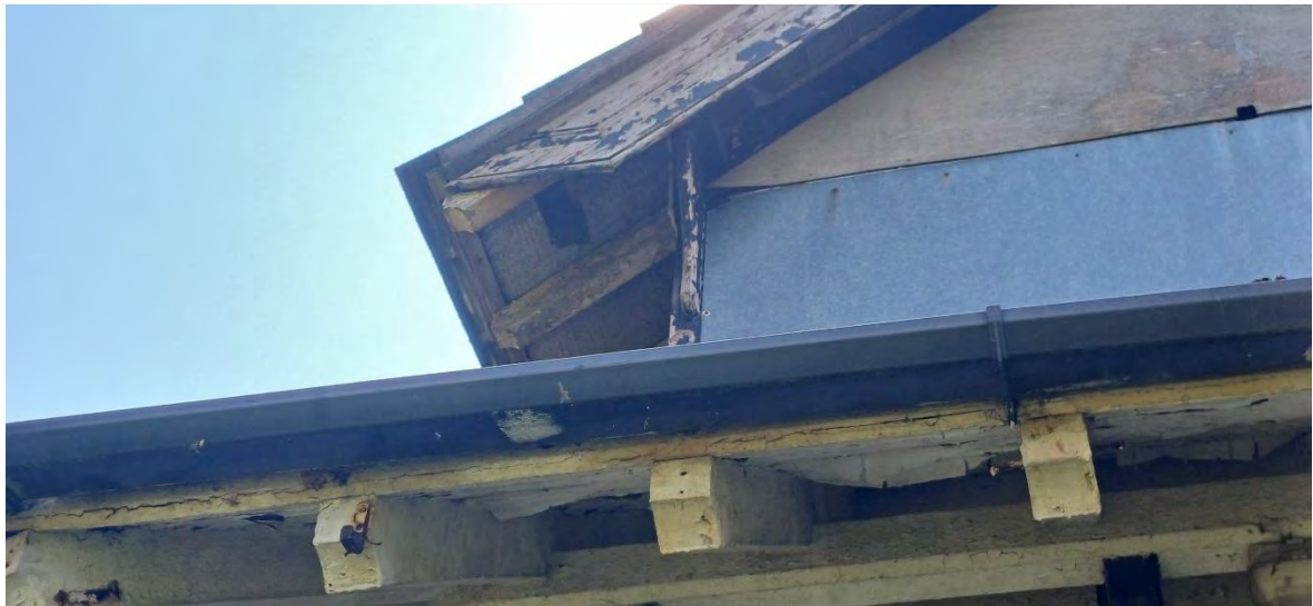
Figure 30 – Right dormer to rear
