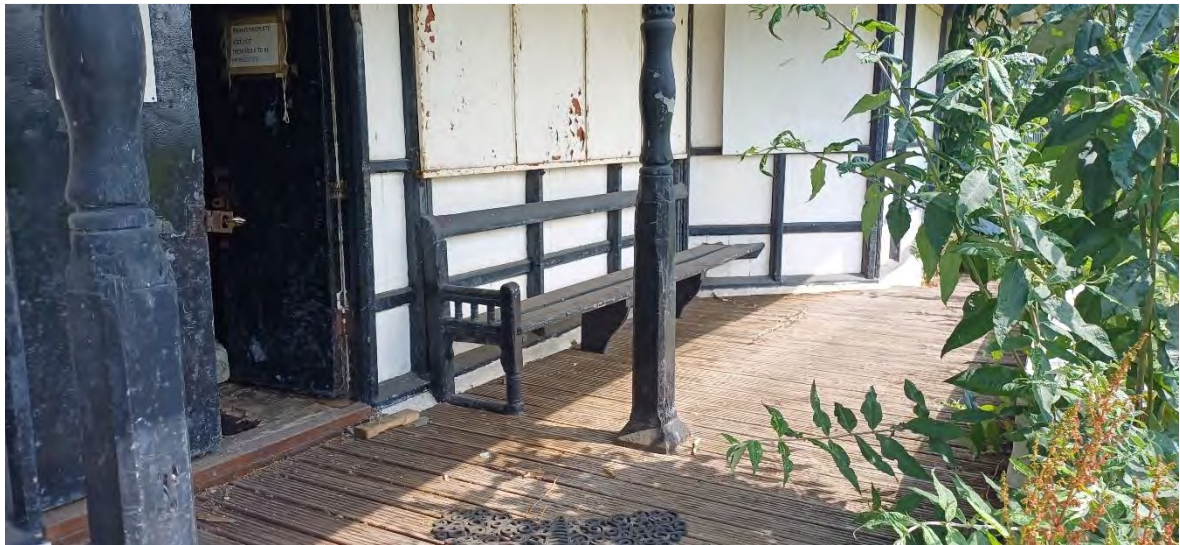
Figure 3 – Timber brackets to roof
