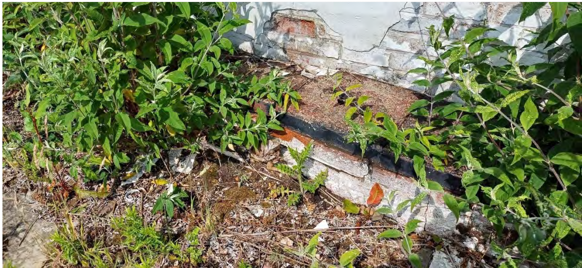
Figure 5 – Retaining wall to veranda
