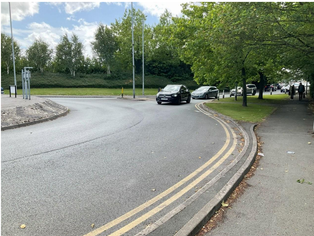
6.2 General view looking south-west from the proposed site access arm.
