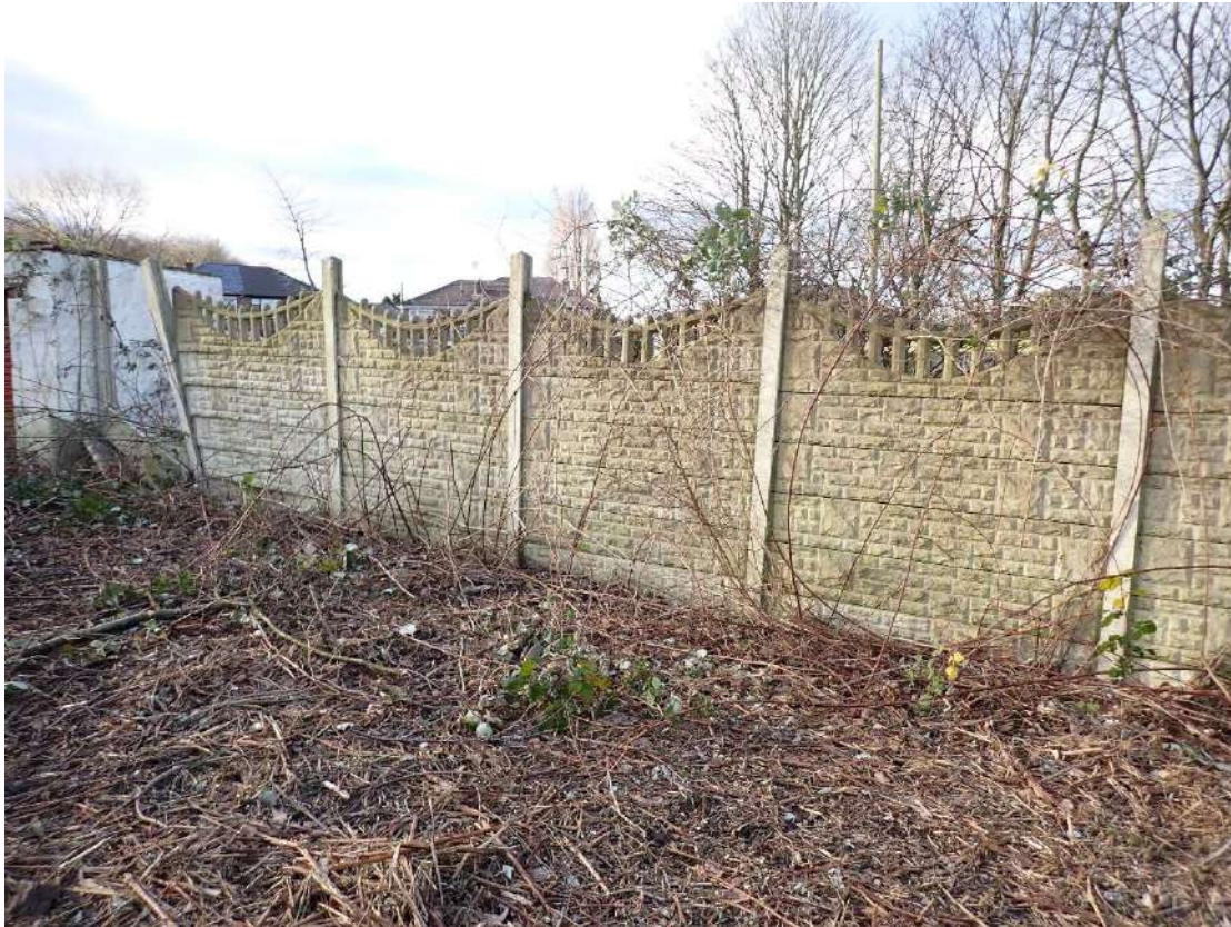
Photograph 17 – Concrete post and panel fencing separating two sections of the proposed development site.
