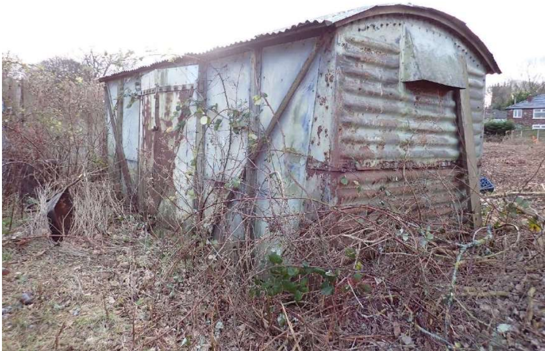
Photograph 13 – A small metal outbuilding (Building 2).
