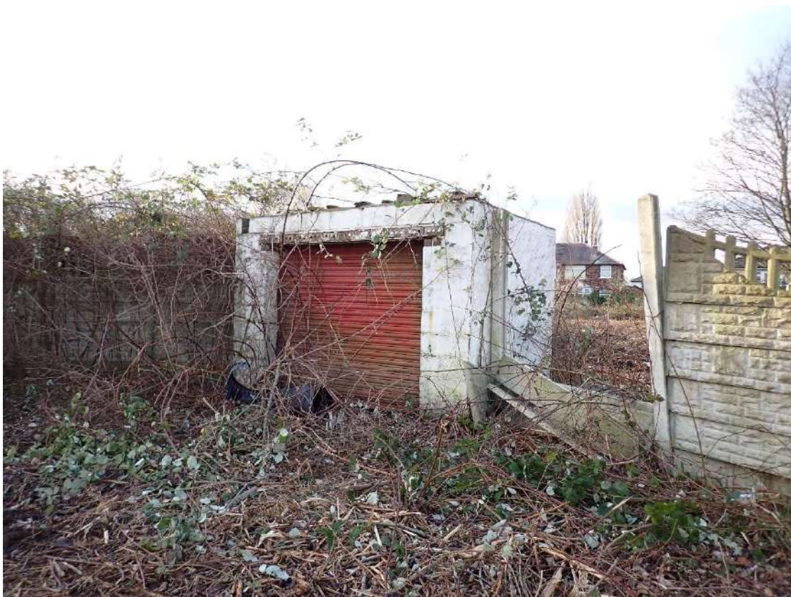
Photograph 14 – A small breezeblock outbuilding (Building 3).
