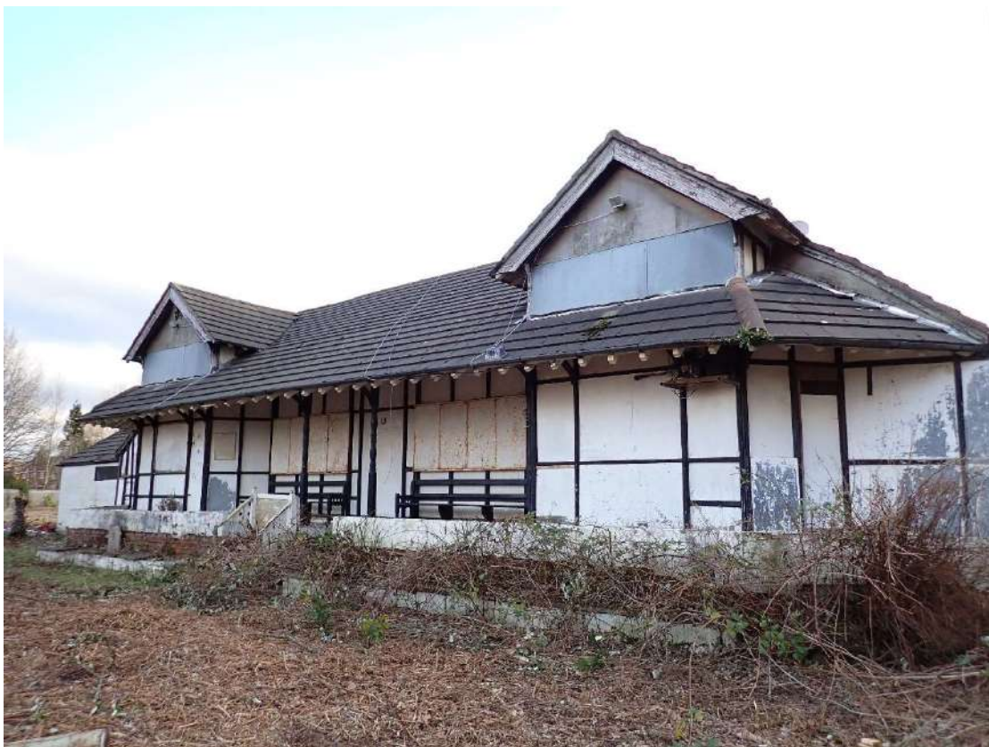
Photograph 12 – The main pavilion building (Building 1).
