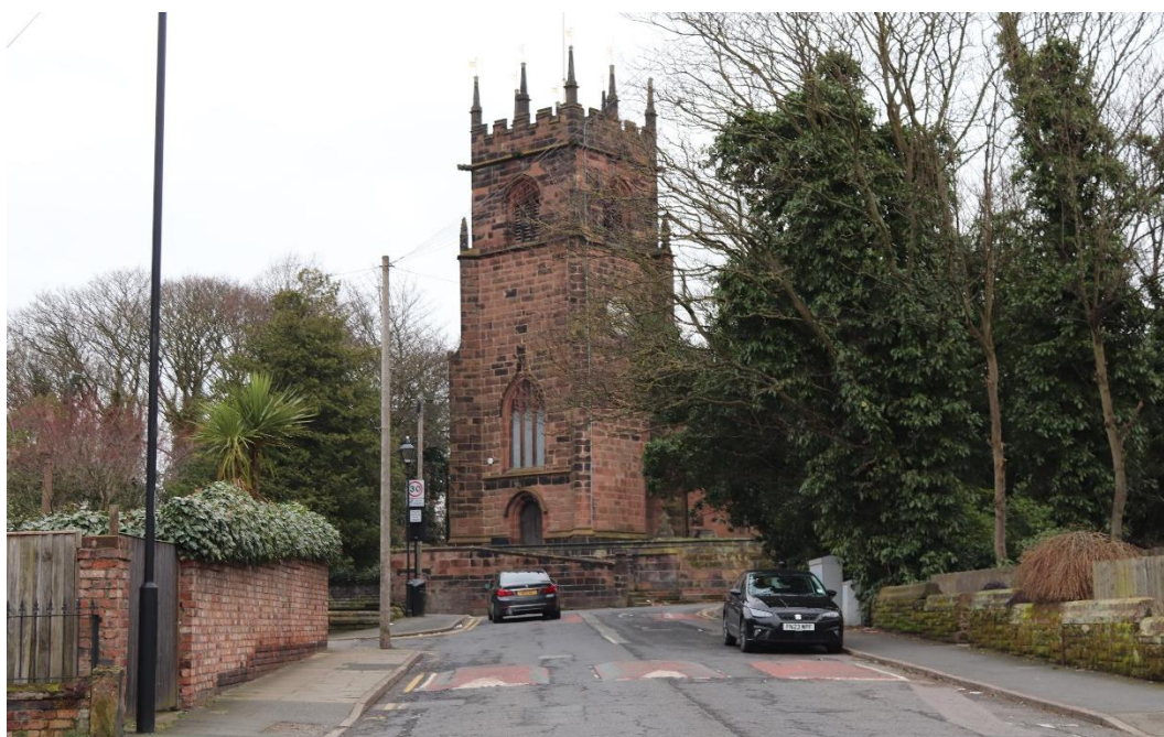
Figure 17: View of Church from Stanley Road
