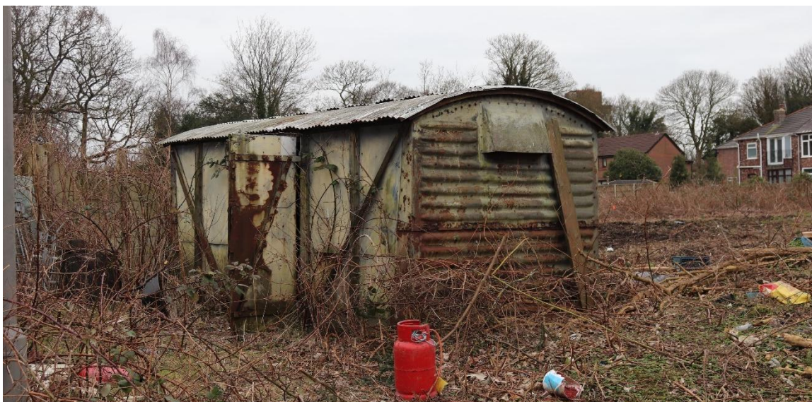
Figure 6: External storage building
