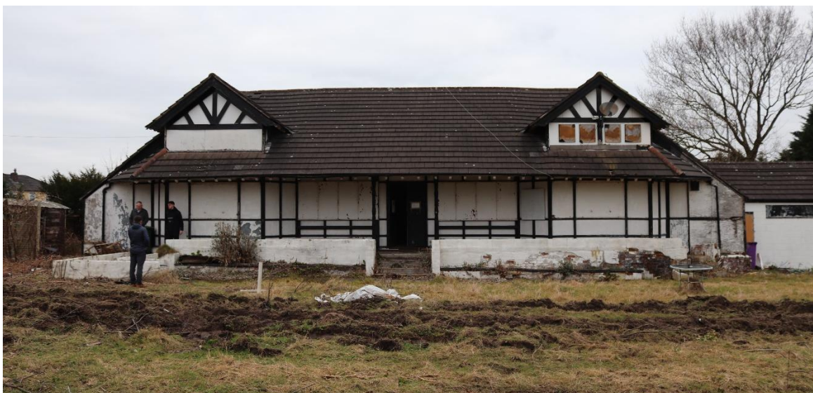
Figure 2: Pavilion, south elevation
