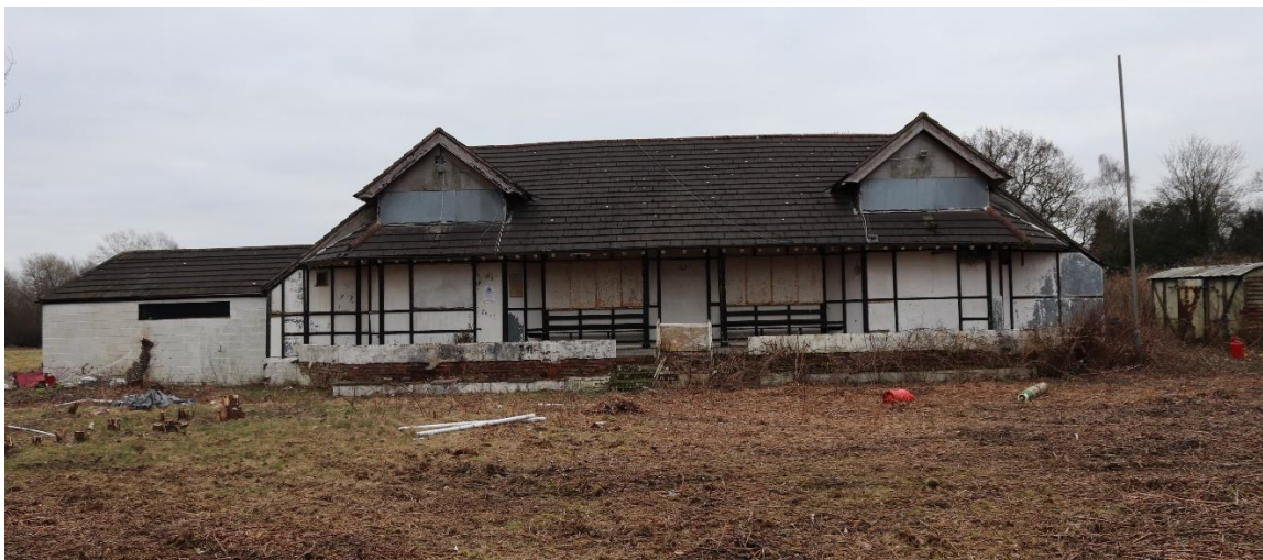
Figure 5: Pavilion, north elevation, viewed from bowling green
