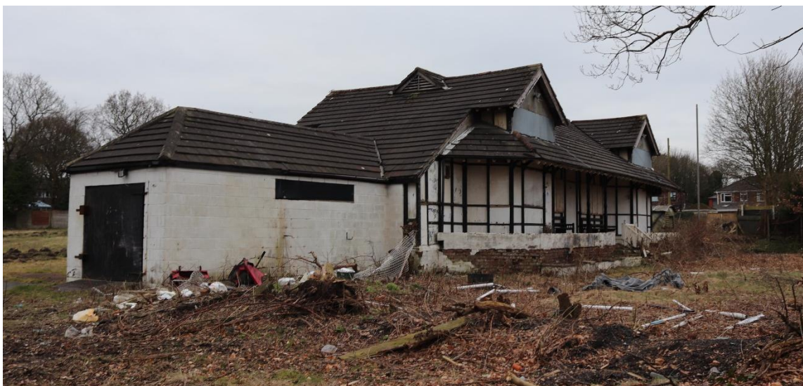
Figure 4: Pavilion, viewed from north-east, showing rear elevation
