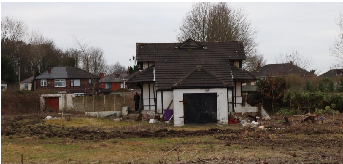
Figure 3: Pavilion, north-east elevation, showing modern extension
