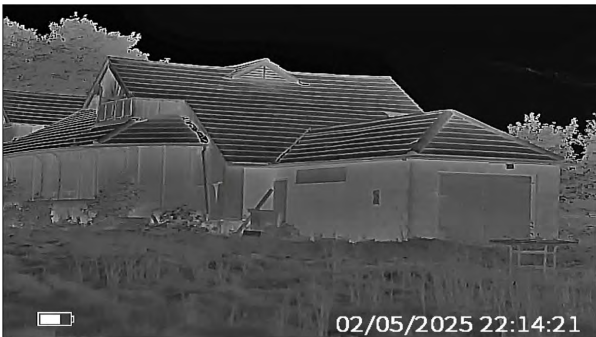
Infrared photograph 4 – Southeastern aspect of Building 1 on 2 nd May 2025.
