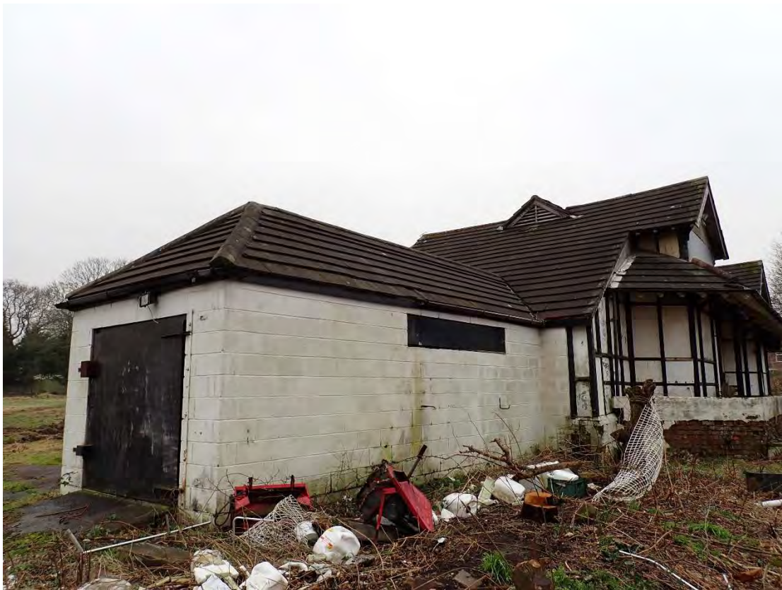
Photograph 2 – Northeastern aspect of Building 1.
