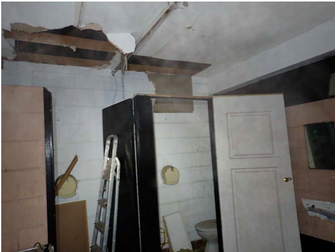
Photograph 16 - Internal space of Building 1.
