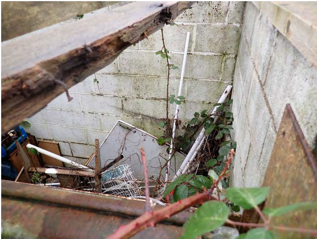
Photograph 20 – Interior of Building 3.
