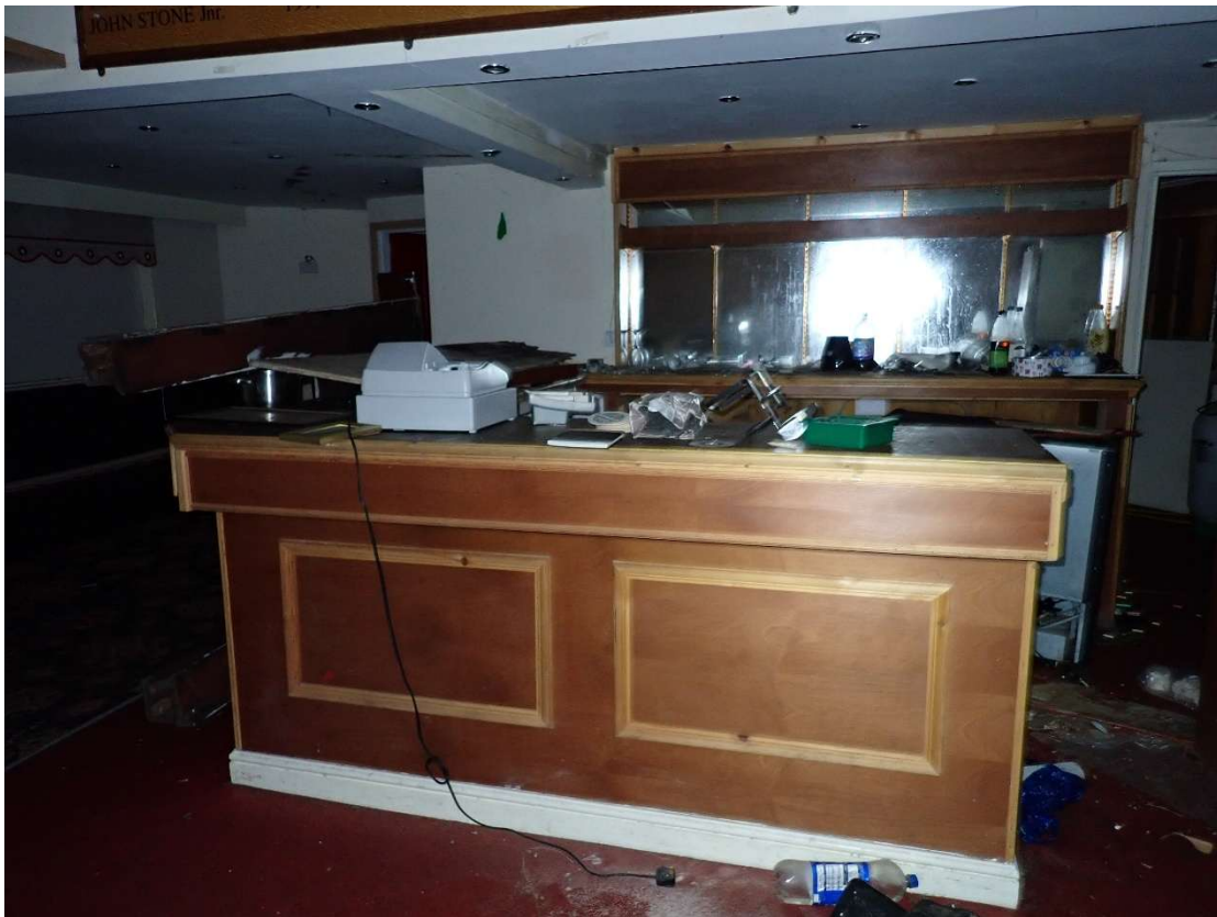
Photograph 18 – Interior of Building 1.
