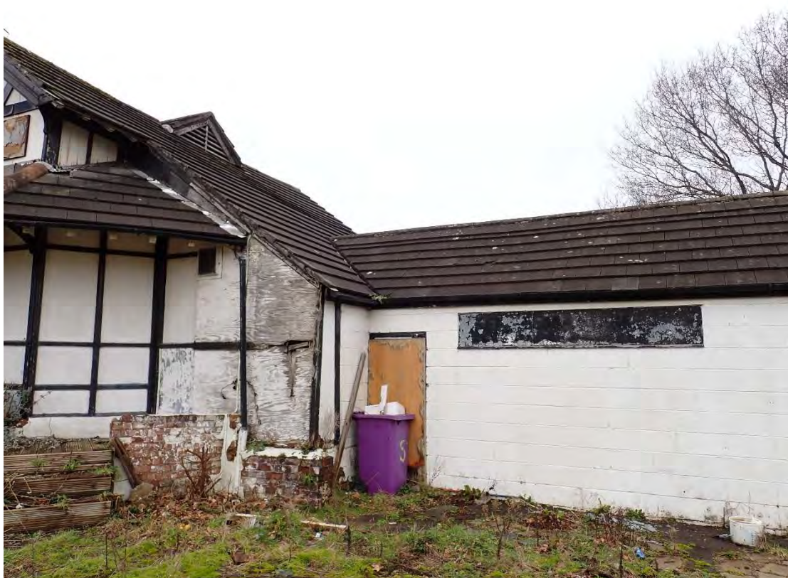
Photograph 3 – Southeastern aspect of Building 1.
