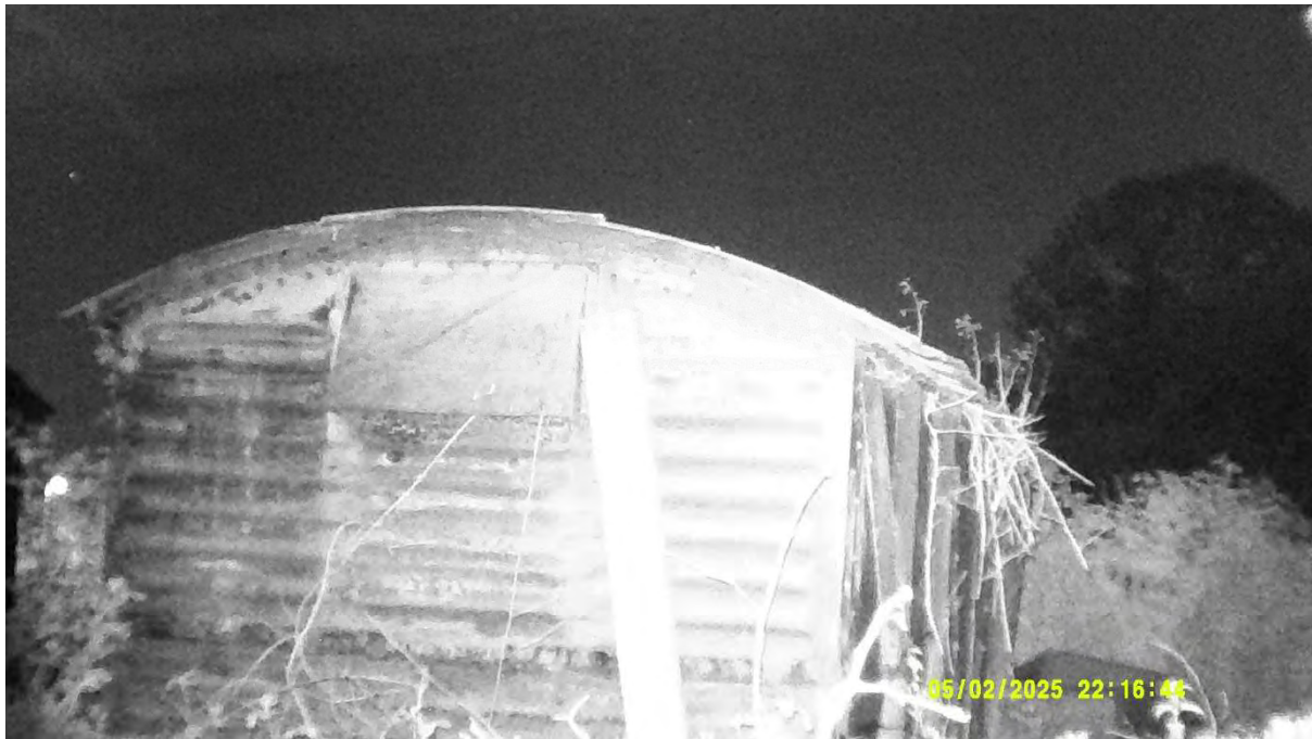
Infrared photograph 1 – Northern aspect of Building 2 on 2 nd May 2025.
