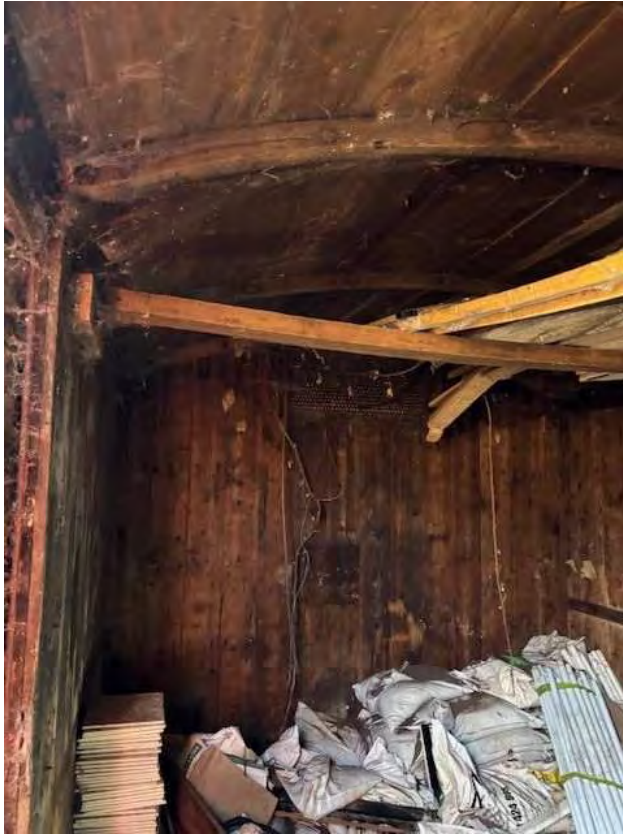
Photograph 19 – The interior of Building 2.
