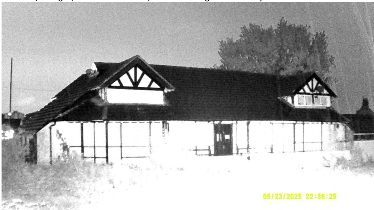
Infrared photograph 6 – Southern aspect of Building 1 on 23 rd May 2025.
