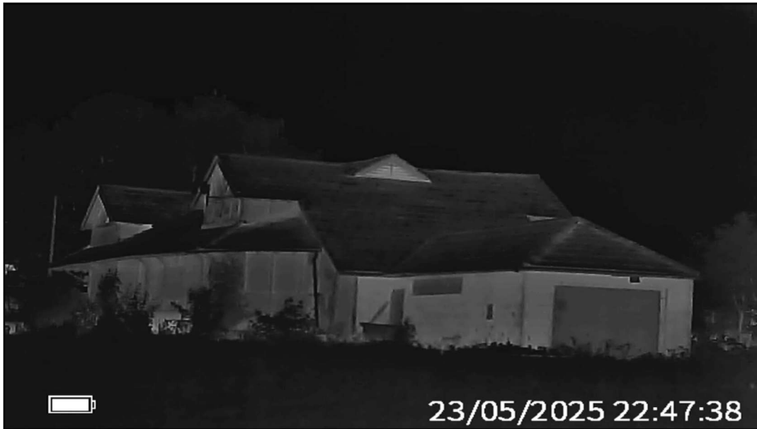
Infrared photograph 9 – Southeastern aspect of Building 1 on 23 rd May 2025.
