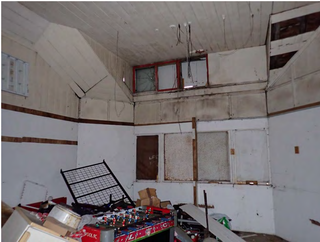
Photograph 15 – Internal space of Building 1.
