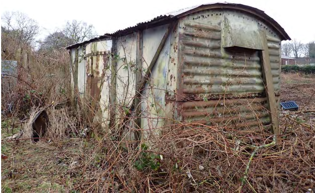
Photograph 9 – Northeastern aspect of Building 2.
