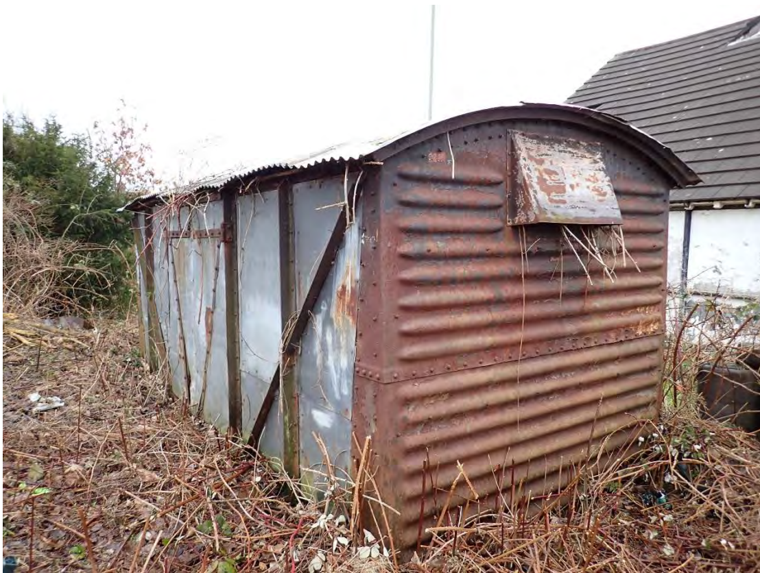
Photograph 8 – Southwestern aspect of Building 2.
