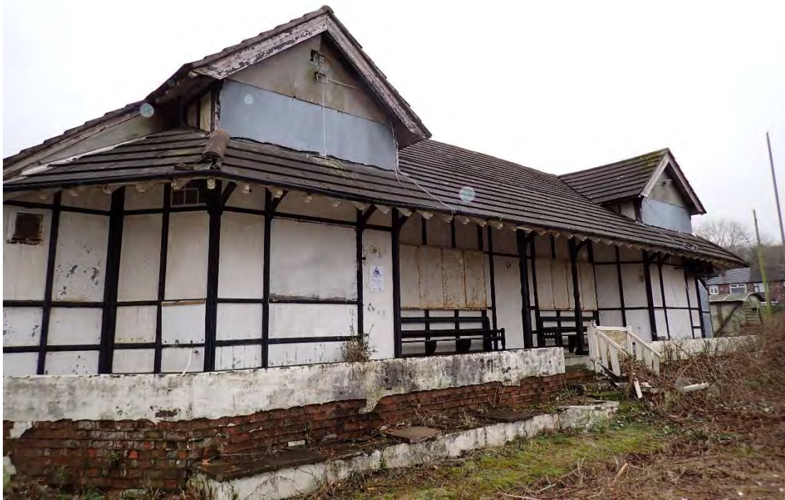
Photograph 1 – Southwestern aspect of Building 1
