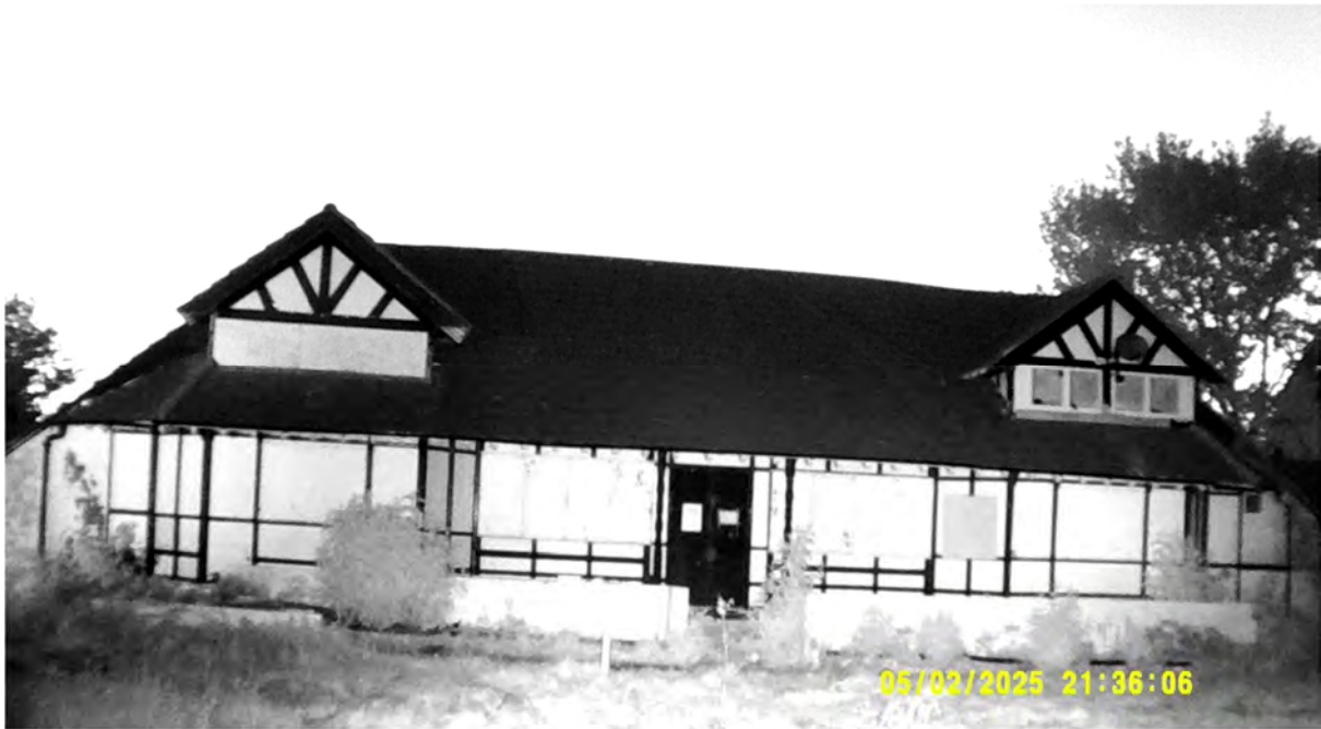
Infrared photograph 5 – Southern aspect of Building 1 on 2 nd May 2025.
