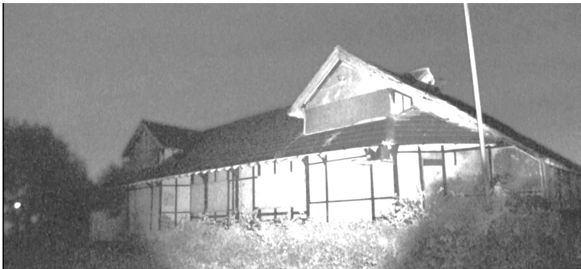
Infrared photograph 8 – Northwestern aspect of Building 1 on 23 rd May 2025.
