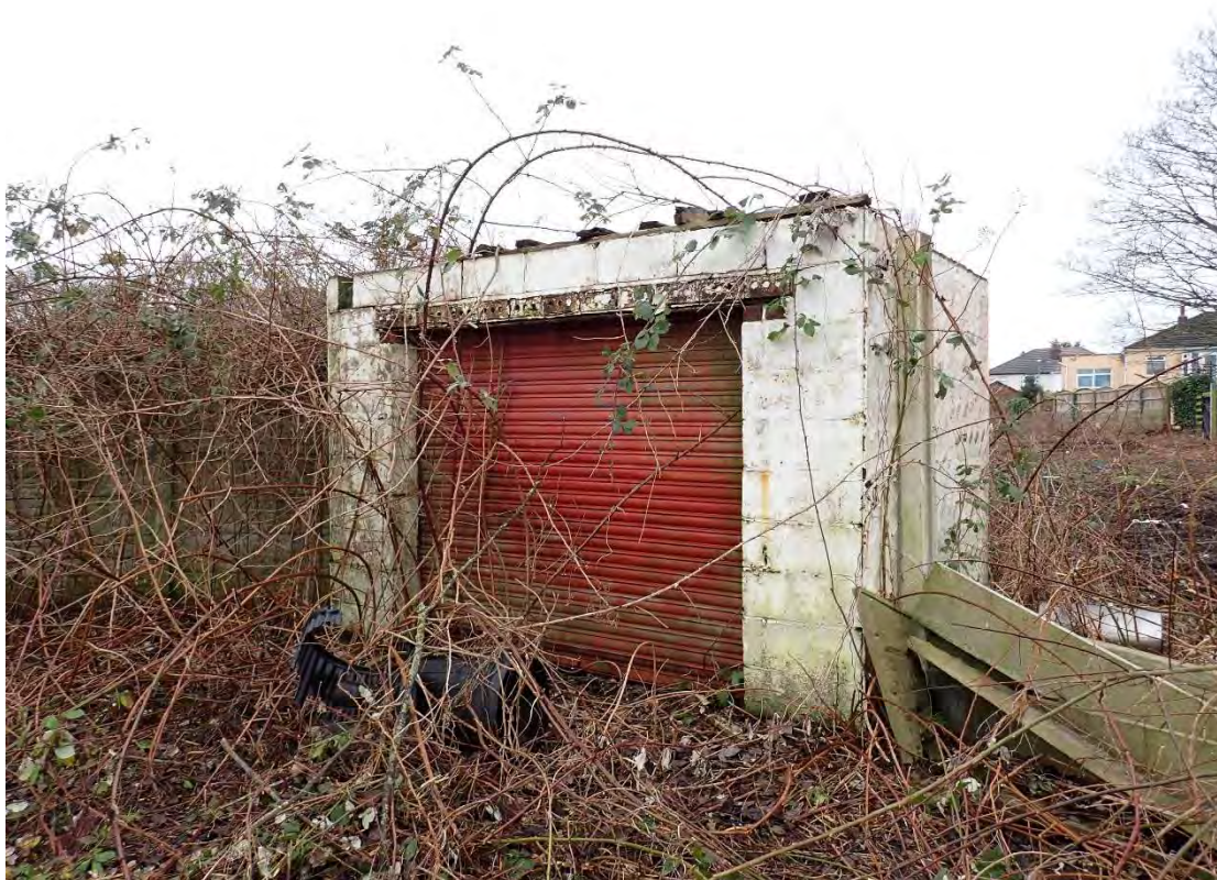
Photograph 11 – The eastern aspect of Building 3.
