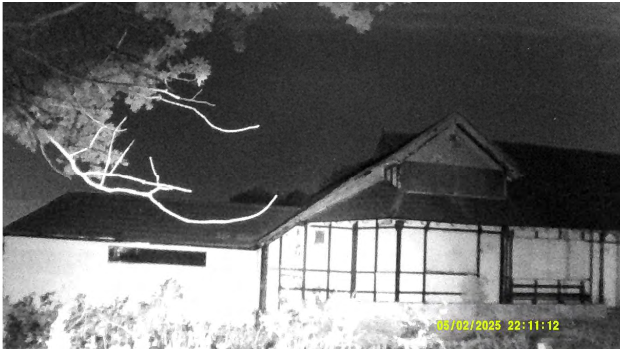
Infrared photograph 3 – Northeastern aspect of Building 1 on 2 nd May 2025.
