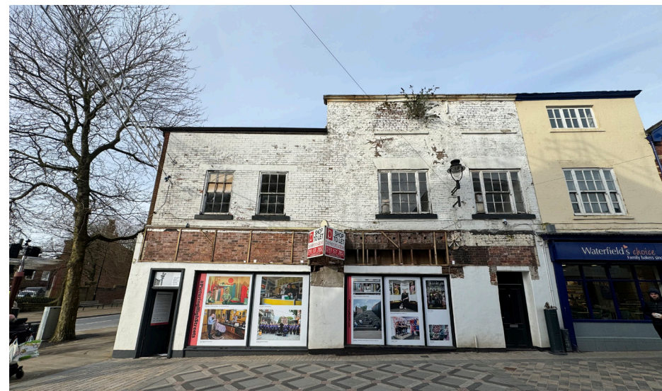
07. View of existing building on site
