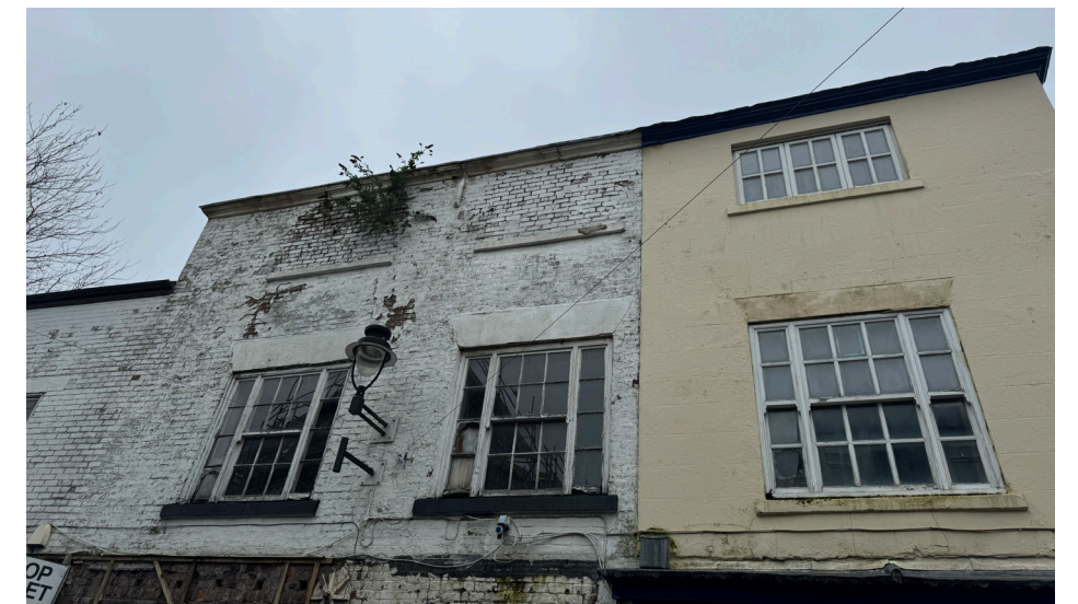
08. View of existing buildings condition
