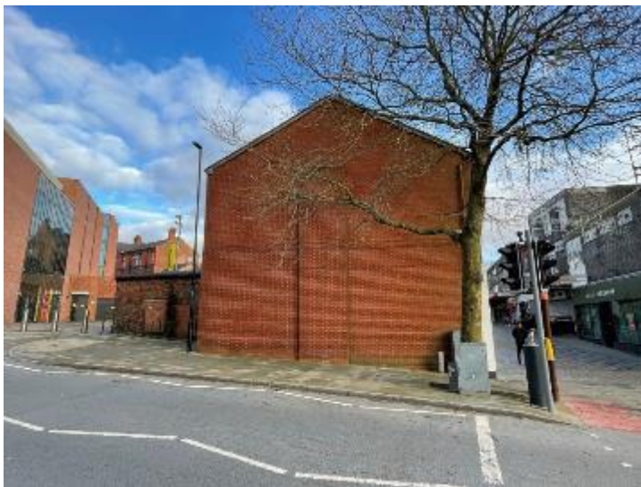
Plate 35: The western elevation of No. 5 Eccleston Street.
