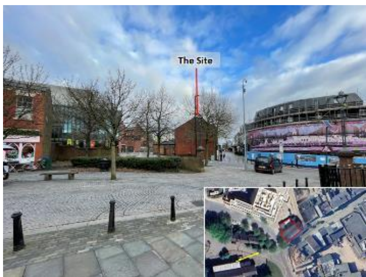
Plate 9: View of the Site from Church Street.
