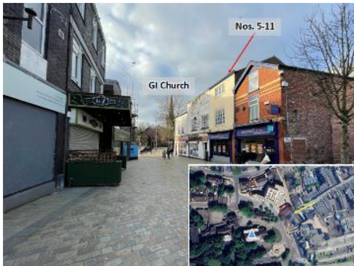
Plate 67: The co-view from Eccleston Street.
