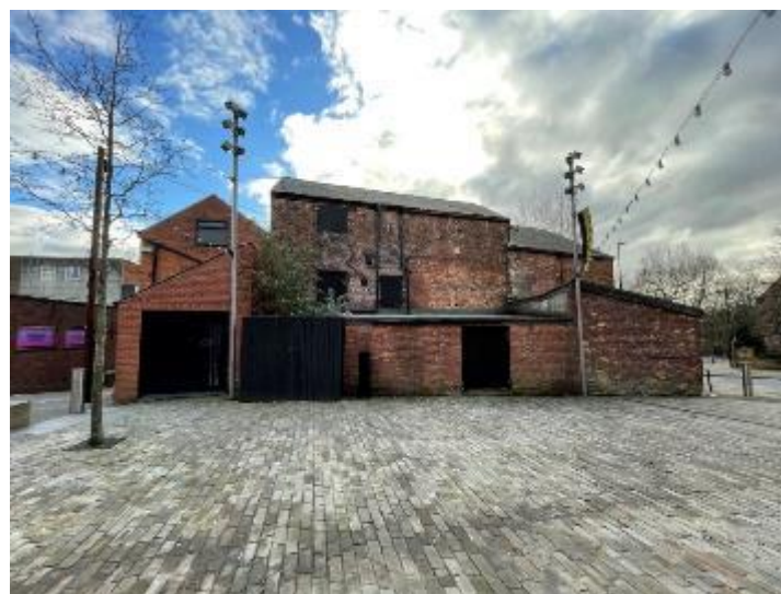
Plate 33: The rear of Nos. 5–11 Eccleston Street.
