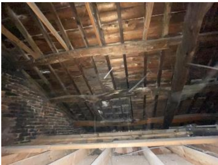
Plate 45: The roof structure within No. 7 Eccleston Street
