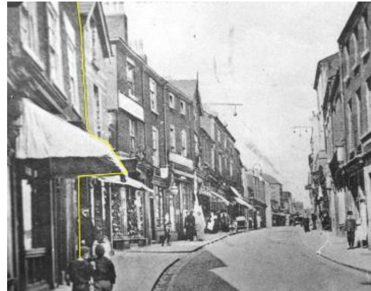
Plate 22: The early 20 th -century photograph of the Site, left of the yellow line, from along Eccleston Street.
