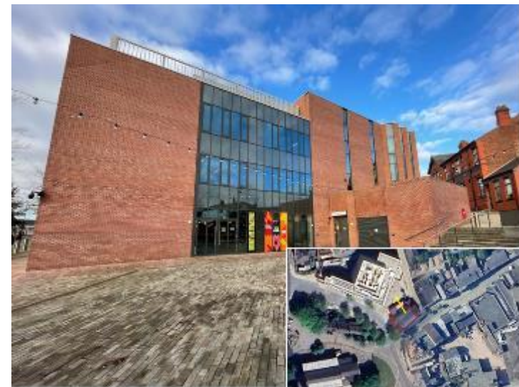
Plate 50: View of the modern yard and playhouse.
