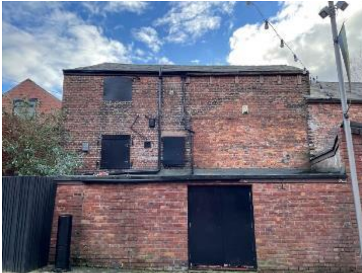
Plate 41: The northern rear elevation of Nos. 7 & 9.
