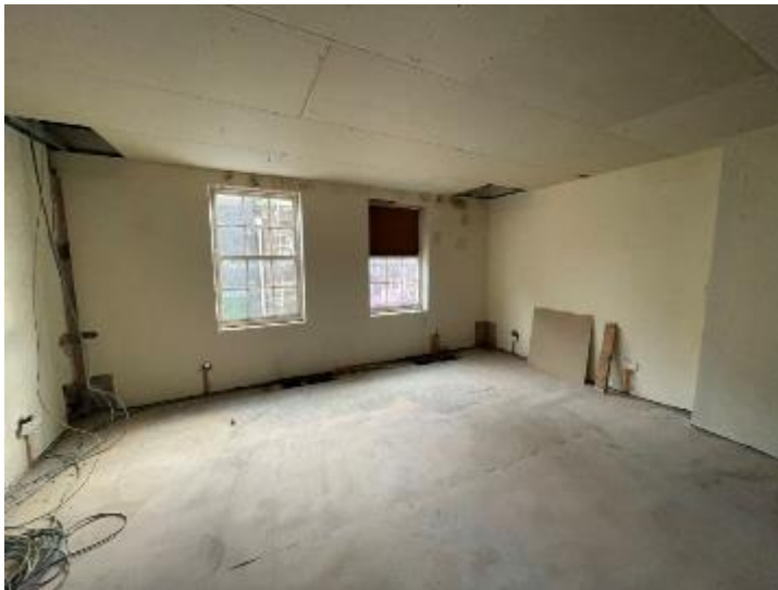
Plate 39: The first floor of No. 5 Eccleston Street.
