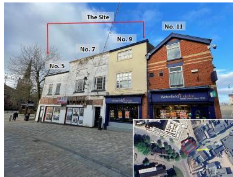
Plate 7: View of the Site buildings from Eccleston Street.
