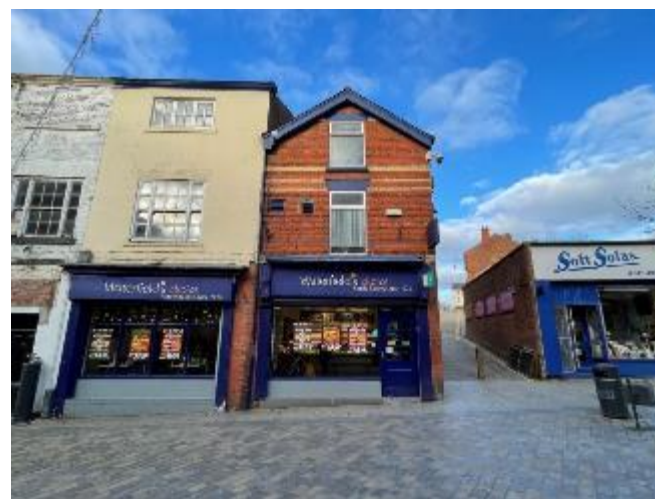
Plate 46: The southern elevation of No. 11.
