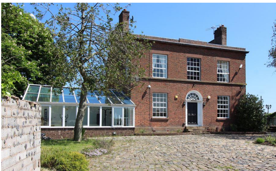
Figure 2: Image showing the front of the property
