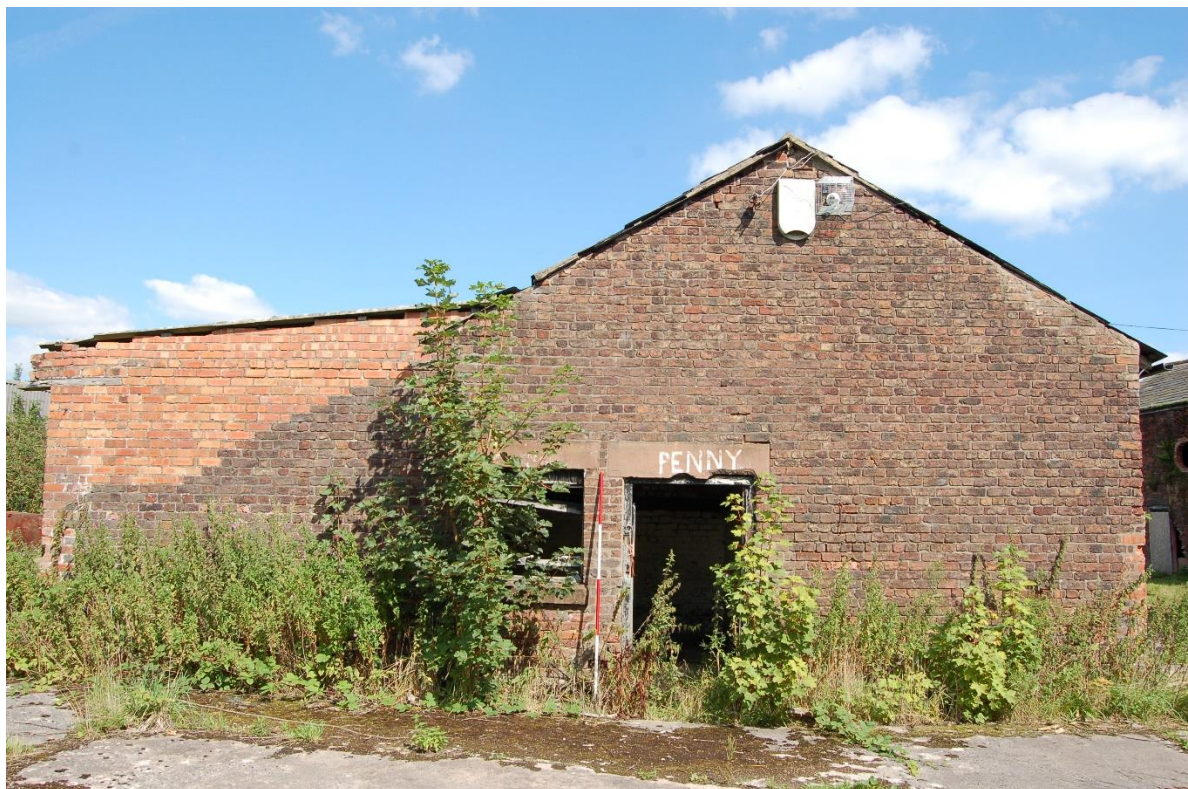
18. West facing elevation of storage barn
