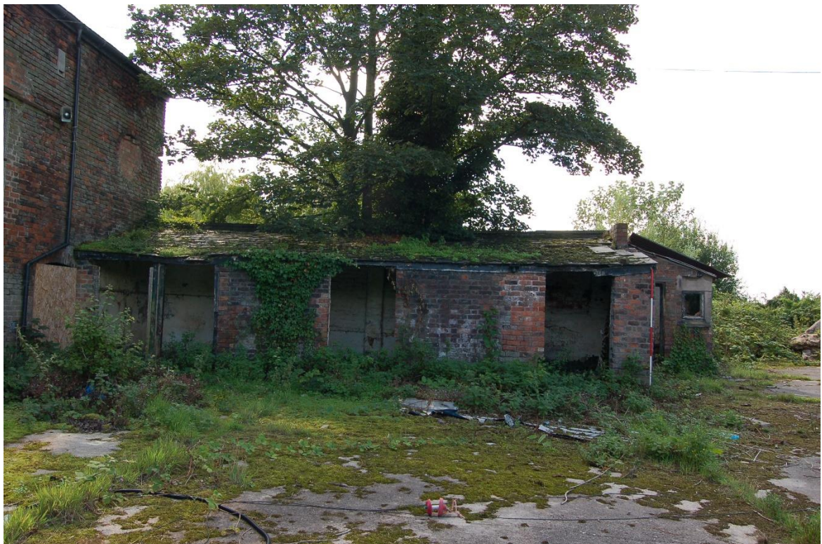
8. Attached barn (north side of main barn) (F8C)
