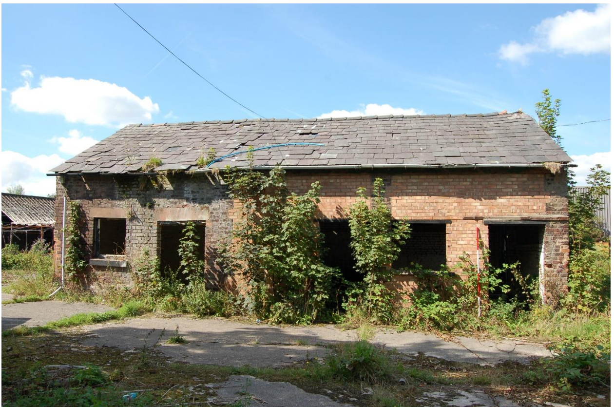
20. South facing elevation of storage barn
