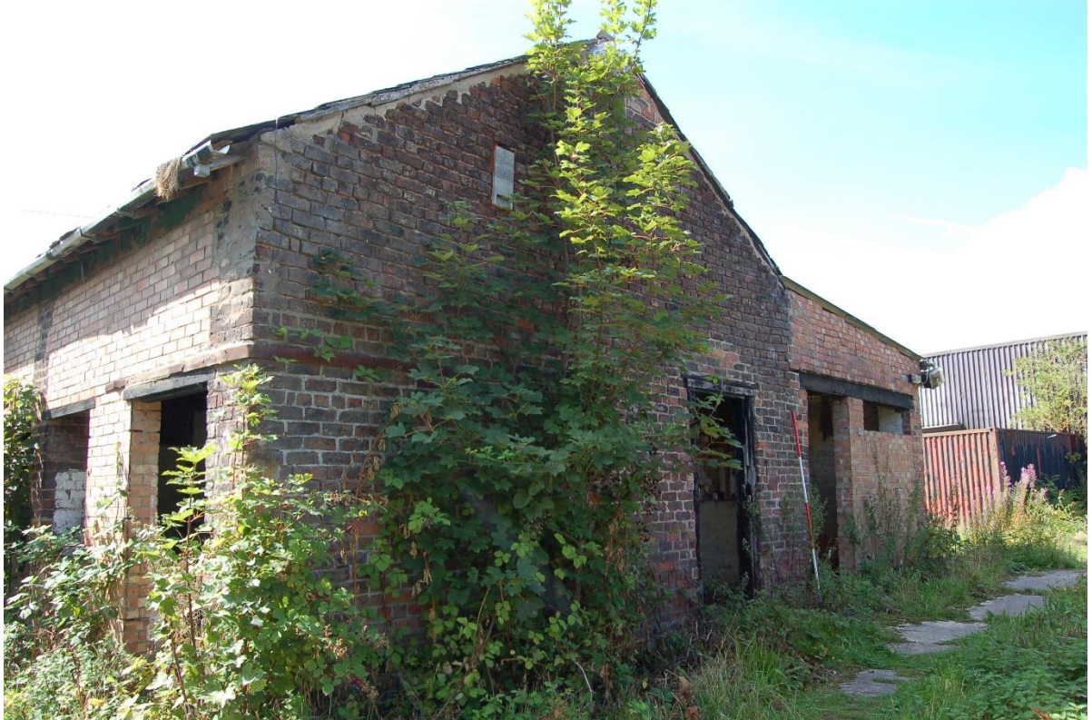
15. East facing elevation of storage barn
