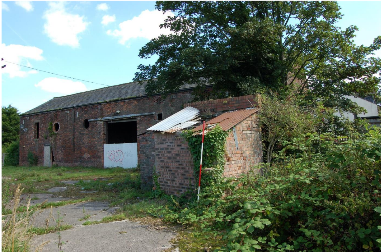
9. Main barn, north facing elevation and northern end of attached barn (F8C)
