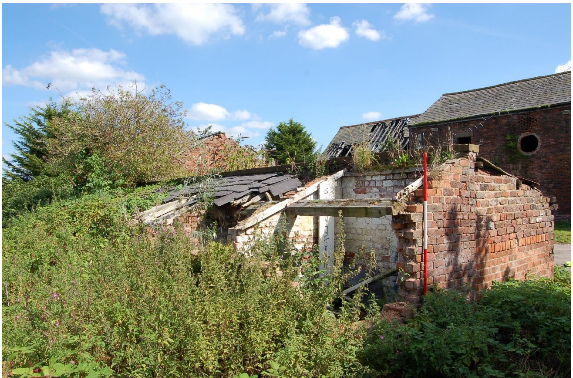
14. West facing elevation of pigsty
