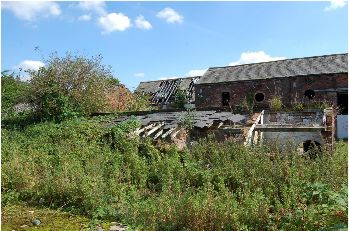
13. North facing elevation of pigsty
