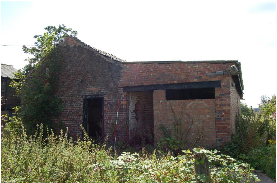
16. East facing elevation of storage barn with modern lean to
